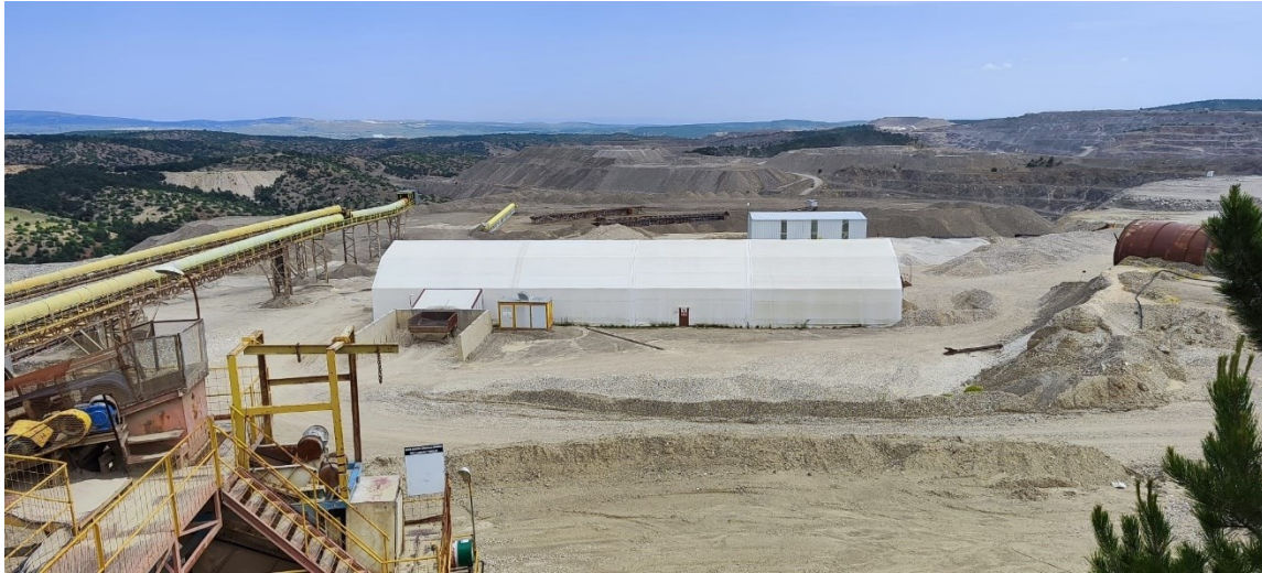
Figure 3-6 Turan tomra facility
