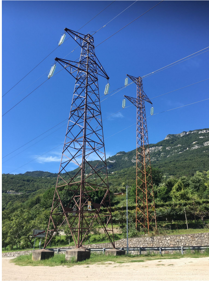
Figure 4.19: Transmission tower used to validate the mapping framework. Following results are referenced to this tower.
