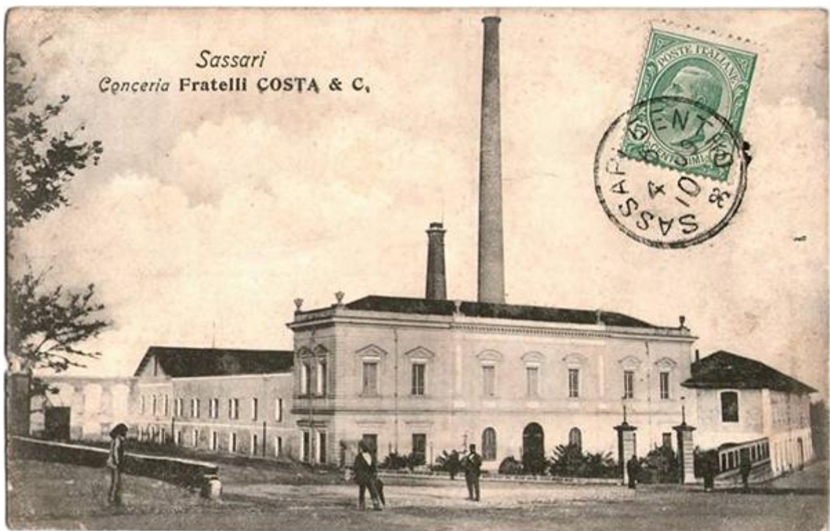
Postcard showing the original aspect of the fabric, first decade XX century
