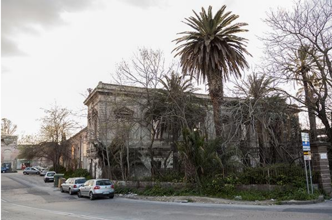
Photography showing the actual aspect of the building after the fire
