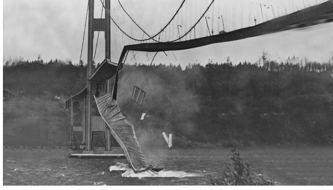
Figure 1.2: Takoma Bridge collapse (source [2]).
