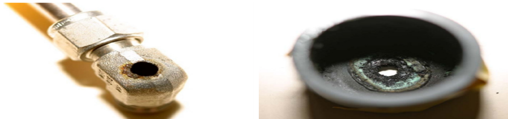
Figure 2.11: Photograph of a stainless-steel fitting and nut drilled by an \text{H}_2/\text{O}_2 flame formed inside the PEM stack adopted [44]
