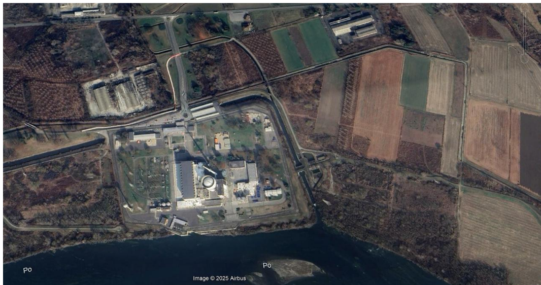
Figure 11 grid infrastructure near the designed solar plant
