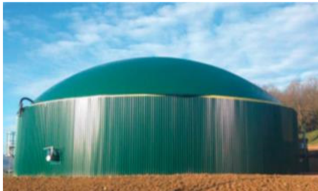
Figure 17 : Example of a double-membrane gasometer dome
