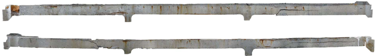
Figure 53: Orthophoto of slab C4
