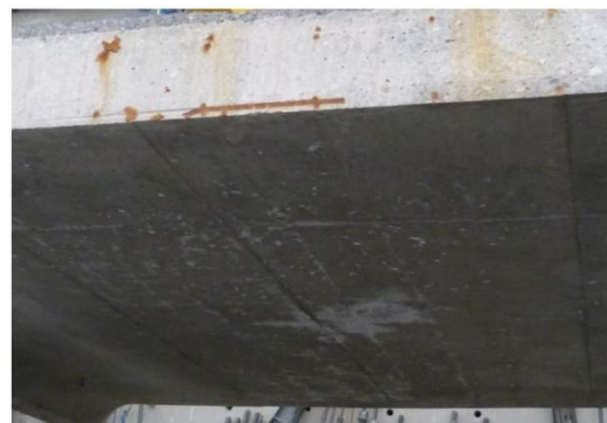
Figure 38: Left: Black spots on span 1. Right: Saline efflorescence on span 2
