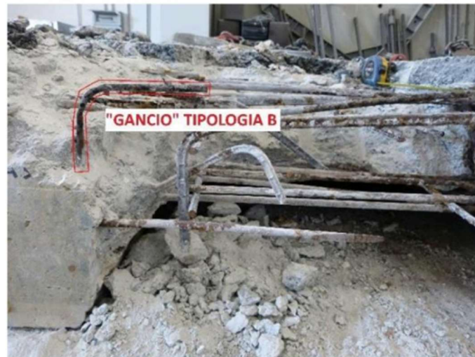
Figure 77: Detail of the hooked bar type B
