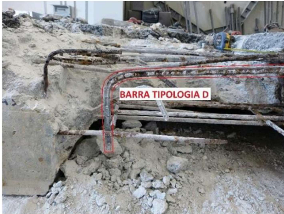
Figure 80: Detail of the hooked bar type D
