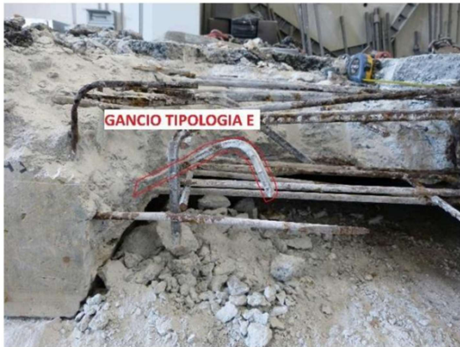
Figure 81: Detail of the hooked bar type E
