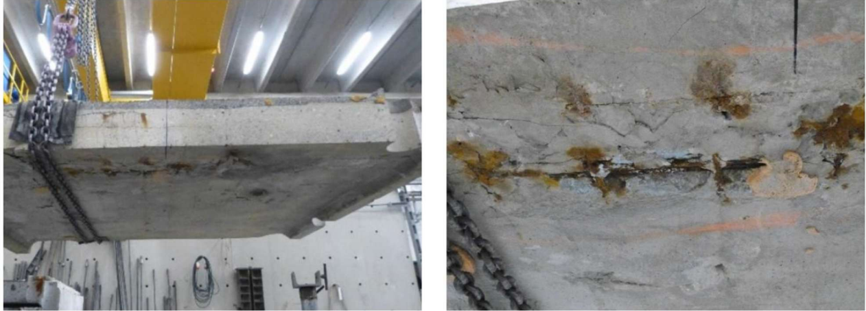
Figure 44: View of small demolition
