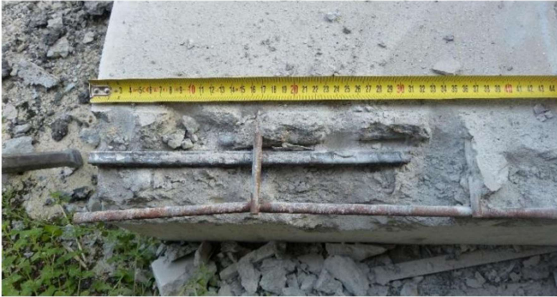
Figure 85: Detail of the bar type F
