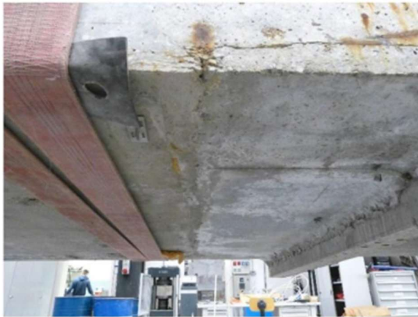
Figure 29: Left: Construction joint between span 2 and span 1. Right: Efflorescence in span 1
