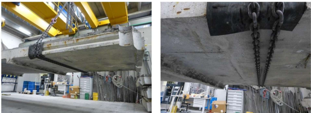
Figure 27: Left: View of span 3. Right: Construction joint between span 2 and 3
