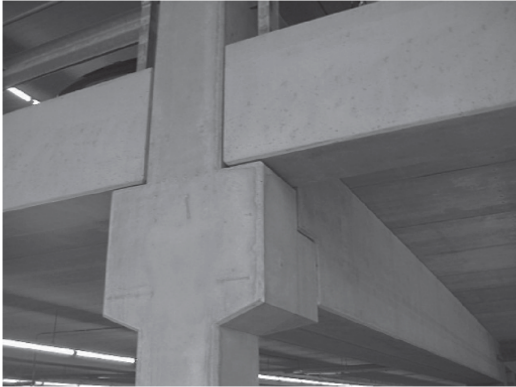
Figure 2 Simple bearing nib and corbel.
