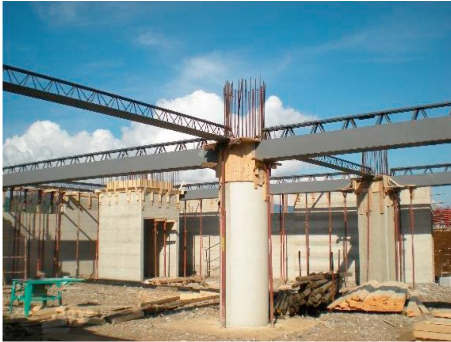
Figure 78 Picture from construction site that highlights the absence of formworks resulting in great cleanliness.
