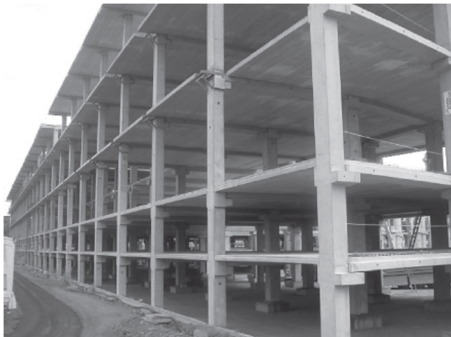
Figure 7 Precast concrete “skeletal” sway frame, Europark, Rome.
