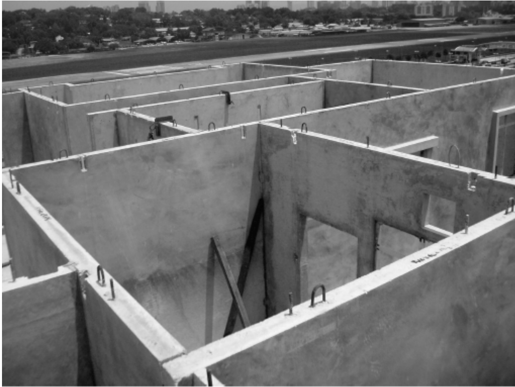
Figure 25 Cross-wall system in precast wall frames.
