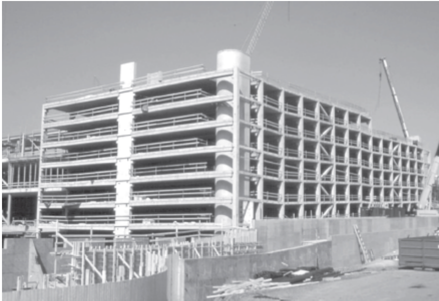
Figure 6 Precast concrete skeletal braced frame, The “Green Apple” retail centre and car park, Helsinki.
