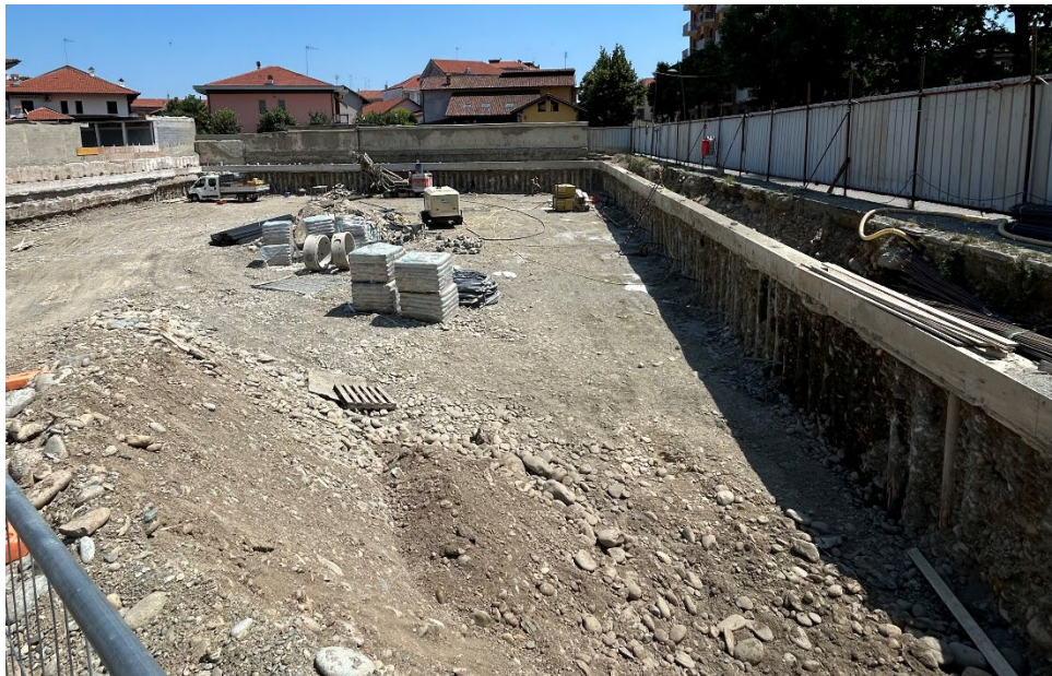
Figure 109 Picture from the construction site showing the micropiles used to stabilise and make safe the excavation process.
