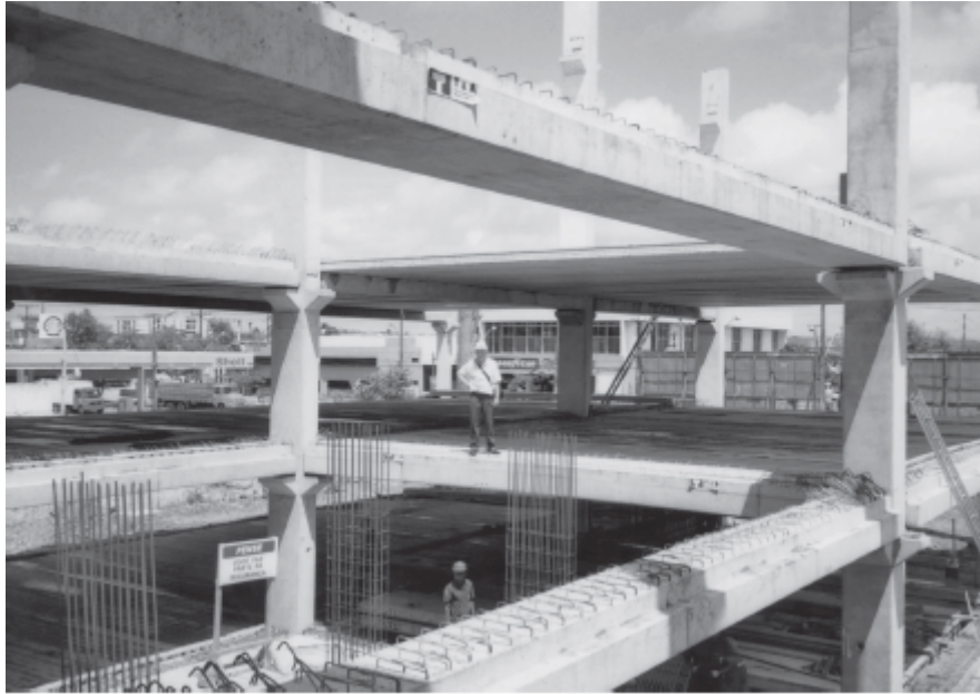
Figure 8 Precast concrete “skeletal” known as “semi-rigid” frame, Recife University, Brazil.
