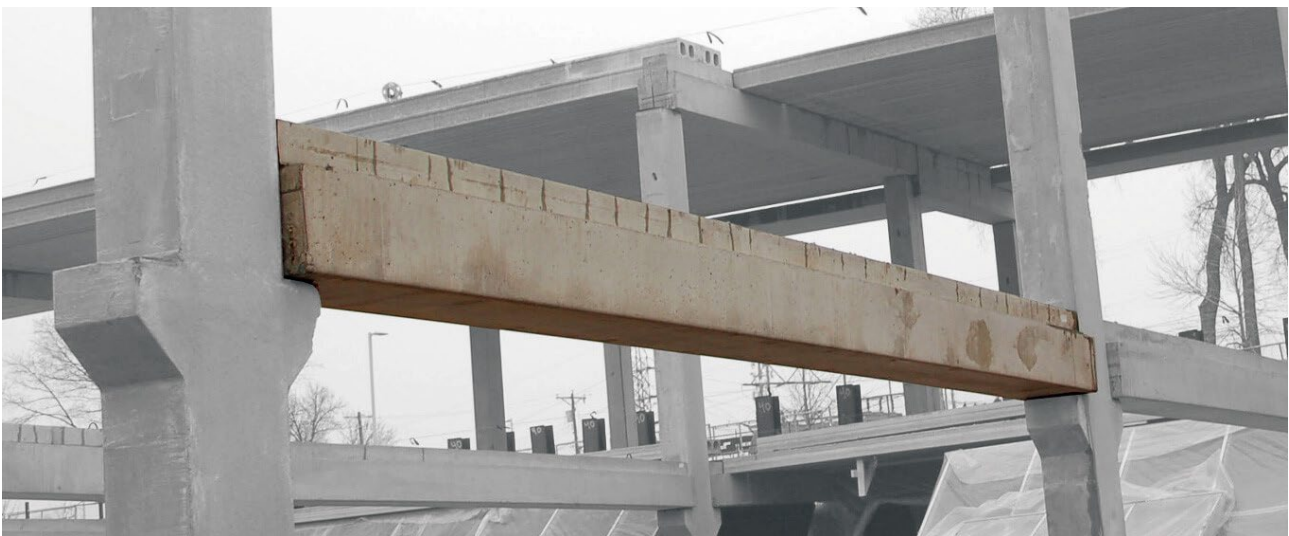
Figure 67 Fully precast concrete beam laying on two precast columns.
