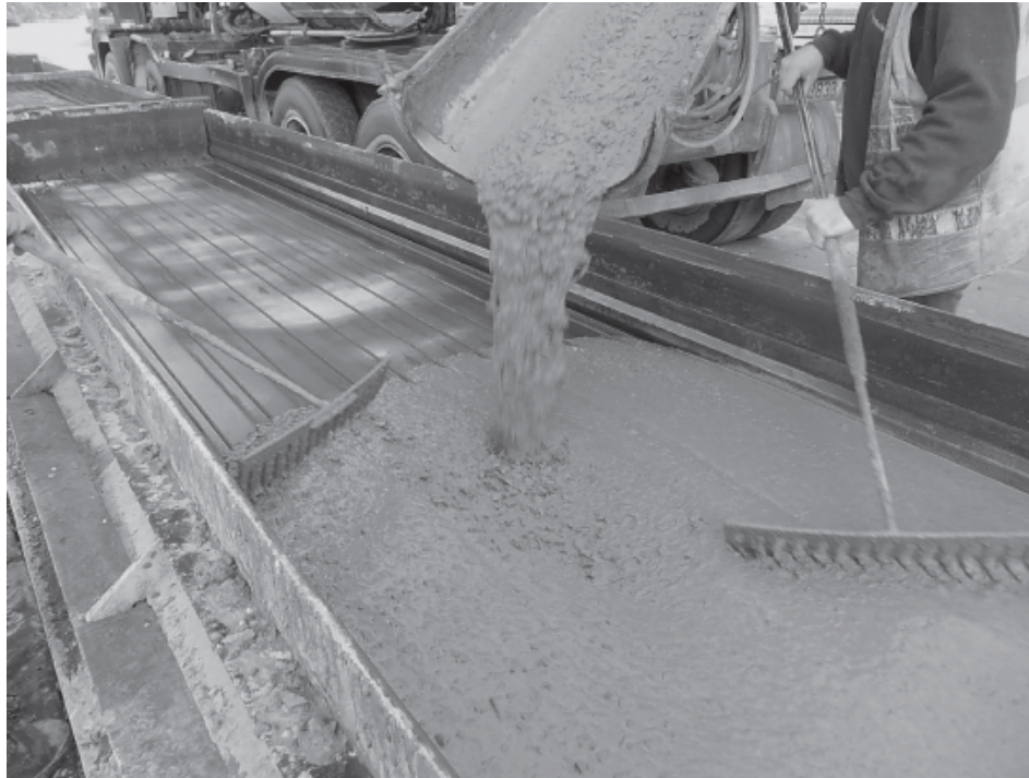
Figure 61 Self-compacting concrete, flowing and compacting without segregation.
