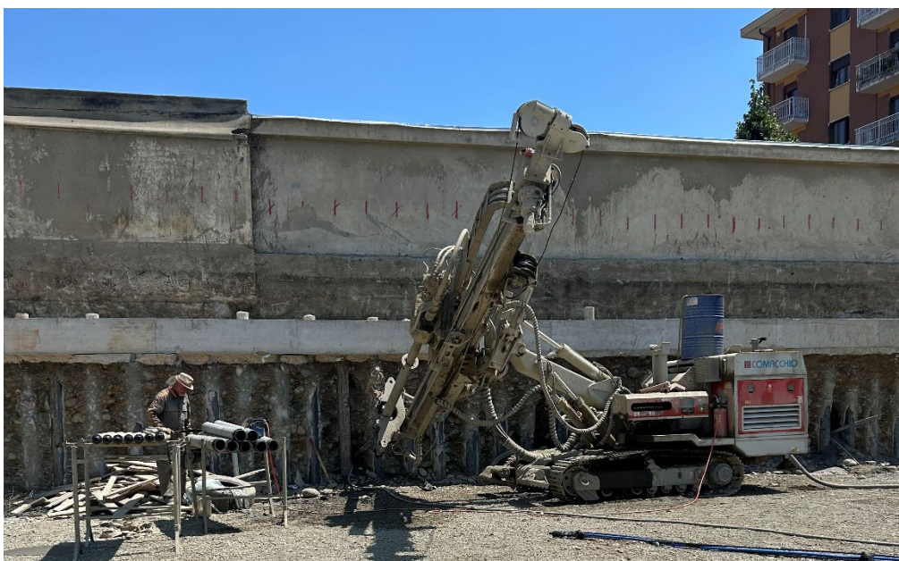
Figure 108 Picture from the construction site showing the drilling machine in action.
