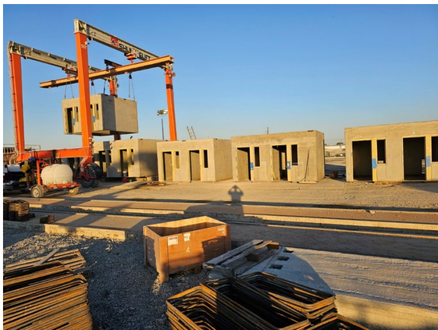
Figure 27 Construction with cell systems moved with a crane.
