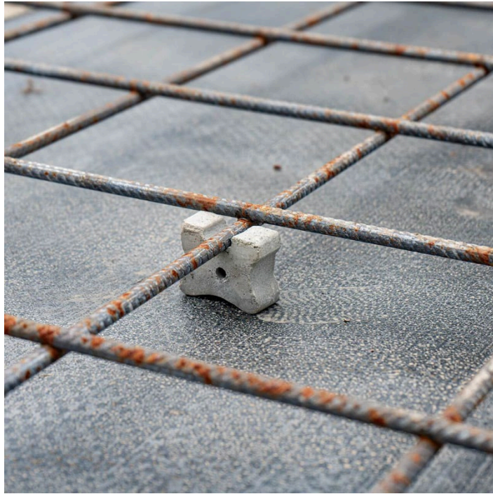
Figure 65 Trestle spacer made in concrete to support horizontal bars.
