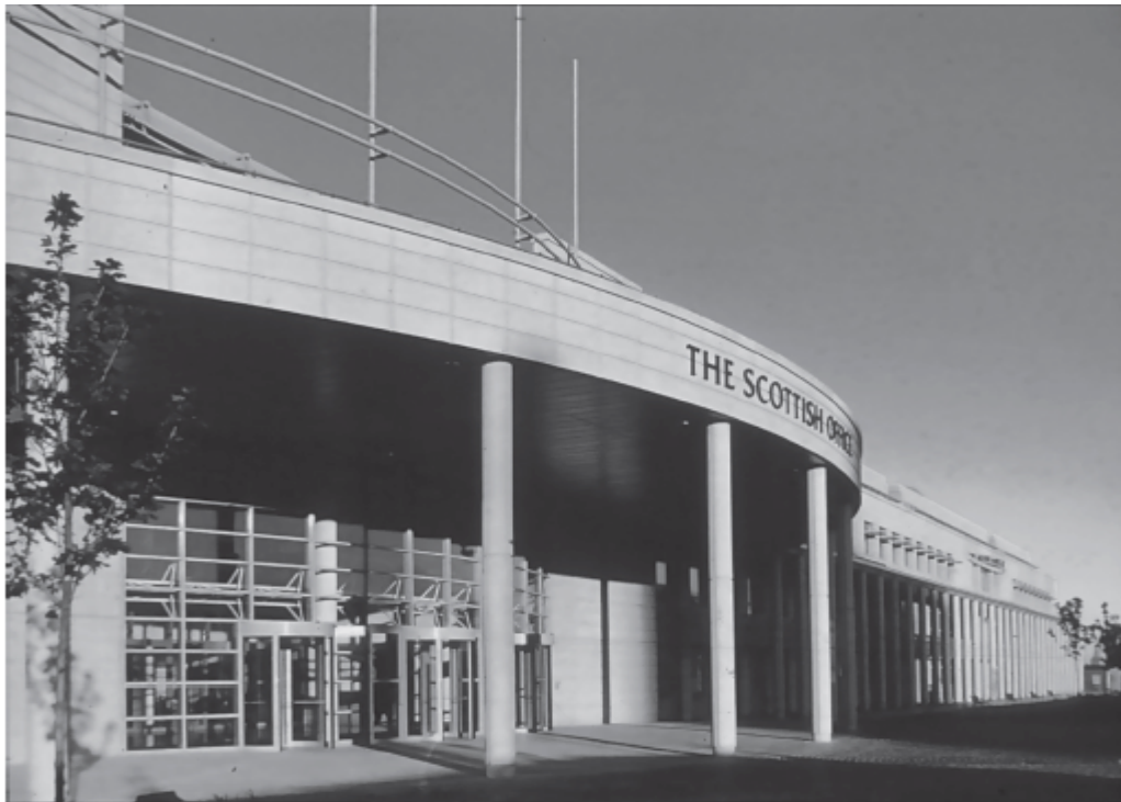
Figure 1 Architectural-structural precast concrete frame at Scottish Office, Leith, United Kingdom.
