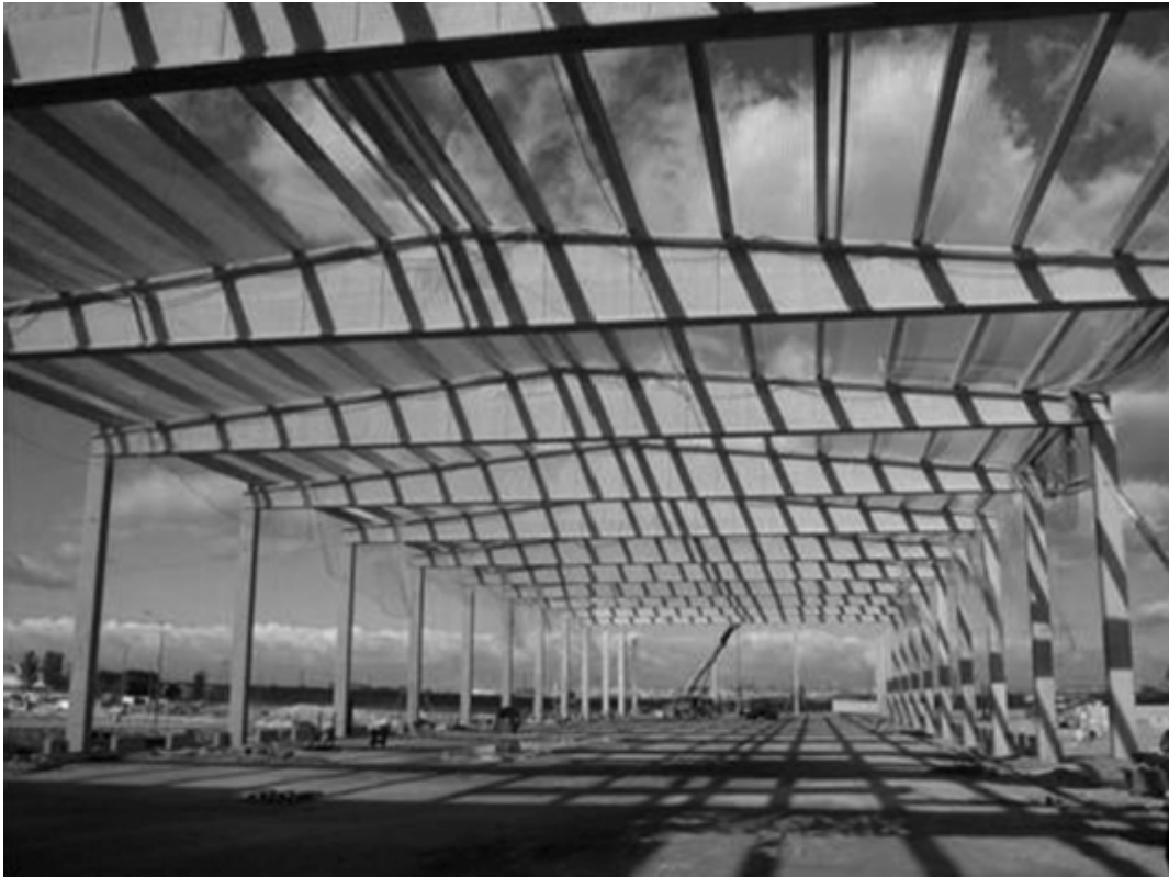
Figure 21 Precast portal frame.
