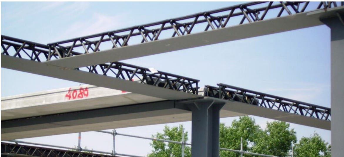
Figure 76 CSTC beams laying into a steel column.
