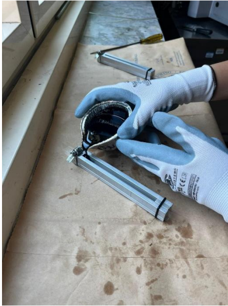
Figure 80 - Pouring bitumen into BBR molds
