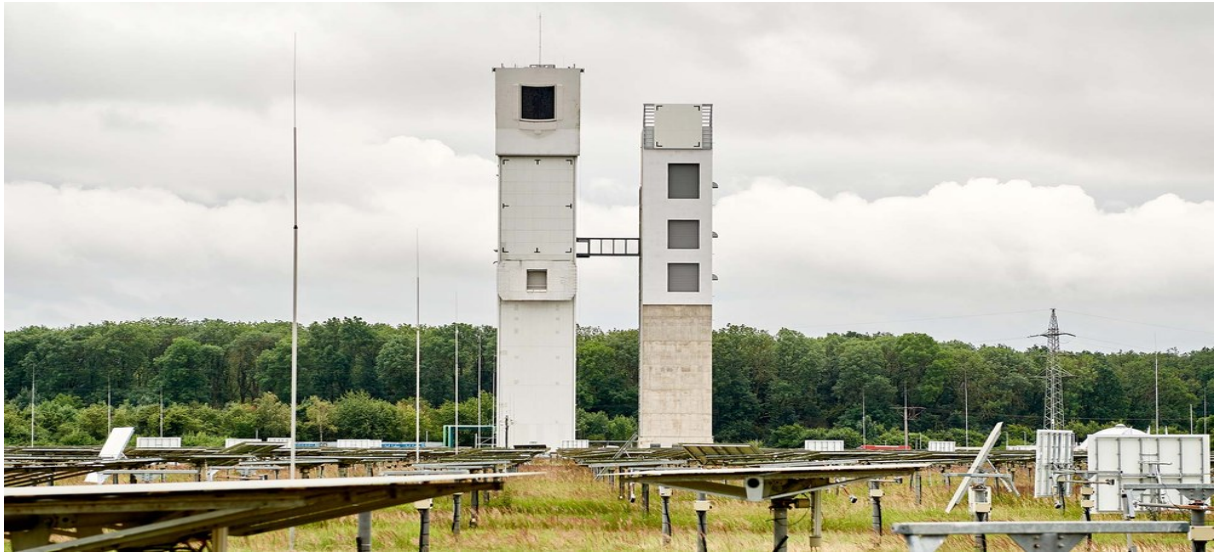
Figure 2.9: The solar thermal tower power plant at DLR Jülich is shown on the left, while the Multifocus Tower, which has been utilized for testing advanced solar technologies since 2020, is on the right[37].
