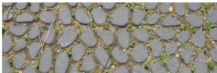
Figure 5.23: Example of permeable pavement [36].
