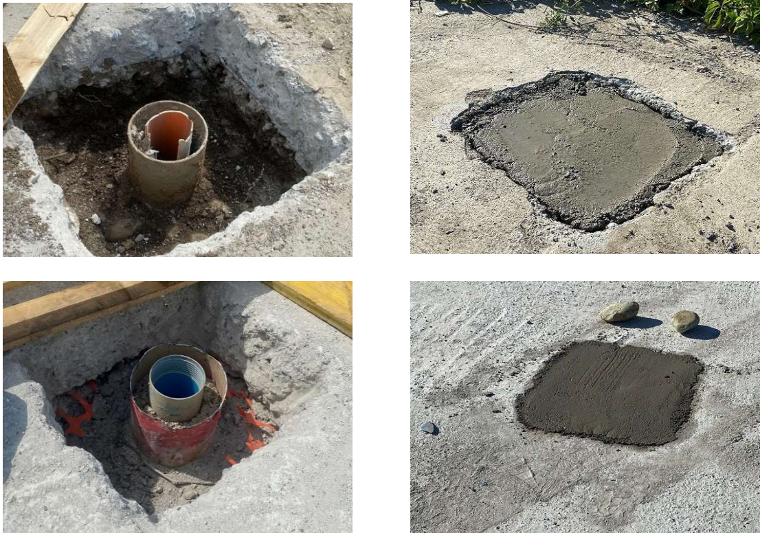
Figure 17. Closure of P2 – above – and P14 – below – piezometers
