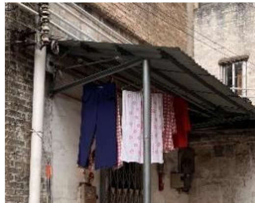
b) Light steel welding
