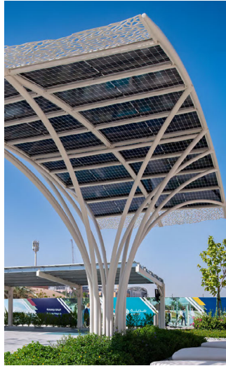
Figure 36 A carport integrated with photovoltaic panels in Masdar City's car park Source: ((Masdar City, 2023b).
