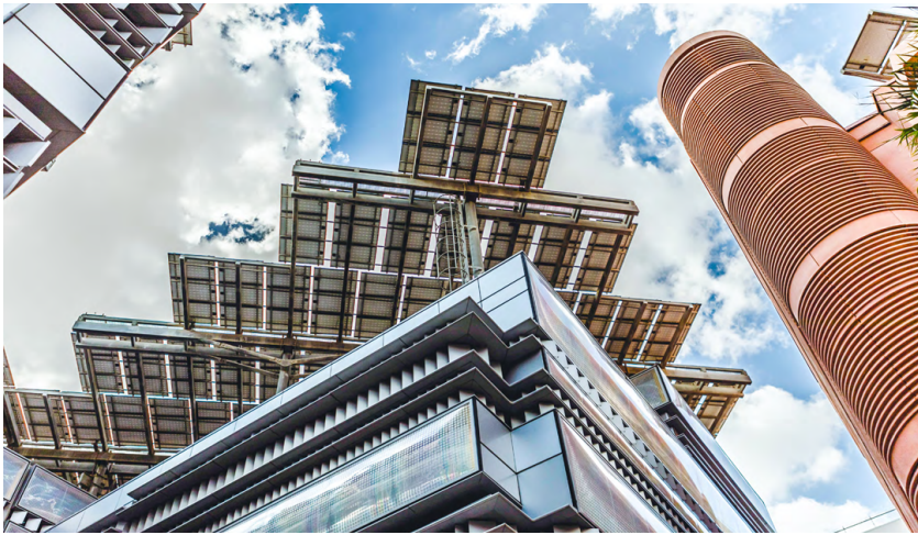
Figure 35 Solar Panel Arrays Mounted Above Building Roofs in Masdar City Source: (Masdar City, n.d.).
