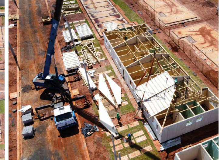
Figure 101: Assemble Different Panels
