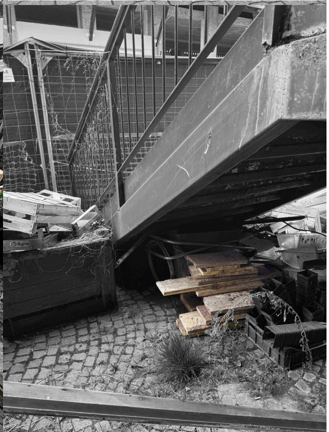
fig 266. Leftover stone pavements, Photo by the author, March 18 2025.
