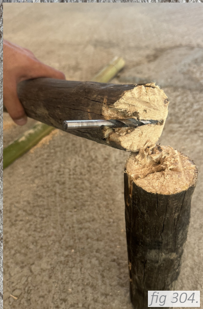
fig 300, 301, 302, 303, 304. Trial of foundation system created by attaching the bamboos to a chestnut tree, with metal screws and drill done by the author, Photos by the author, June 18 2025.
