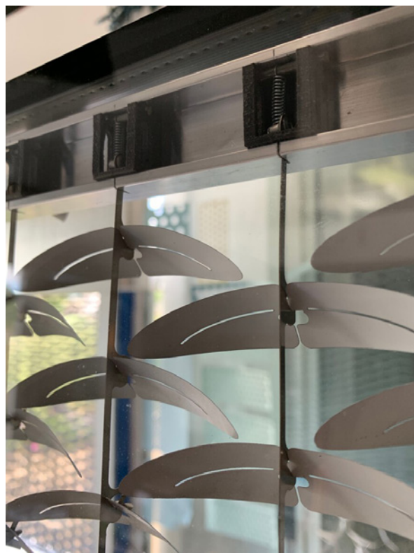
Fig [xv] Detail View of the InVert Panel [34]
