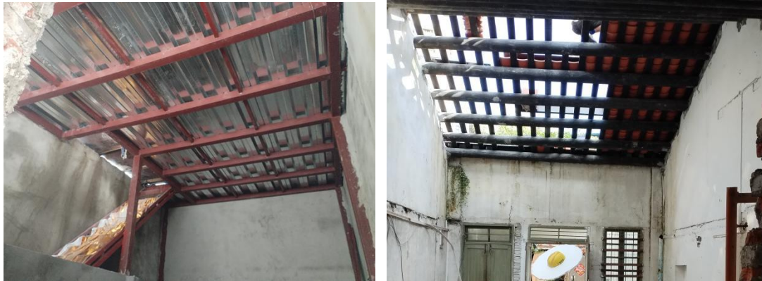
Figure 2.2-17 Left: Roof after steel structure reinforcement Right: Roof during wooden structure repair
