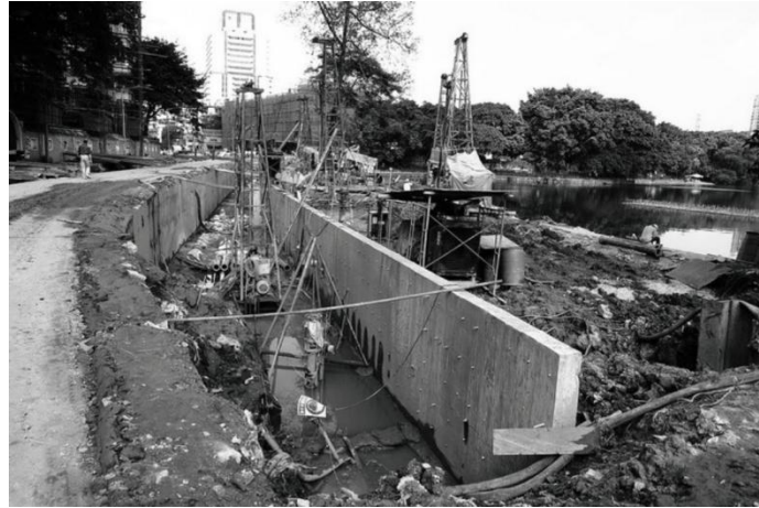
Figure 3.5-5 Photo of the Lizhi River channel being uncovered after re-emergence
