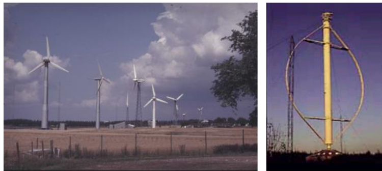
Figure 2.1 :Horizontal axis wind turbines (left) and vertical axis wind turbine (right)
