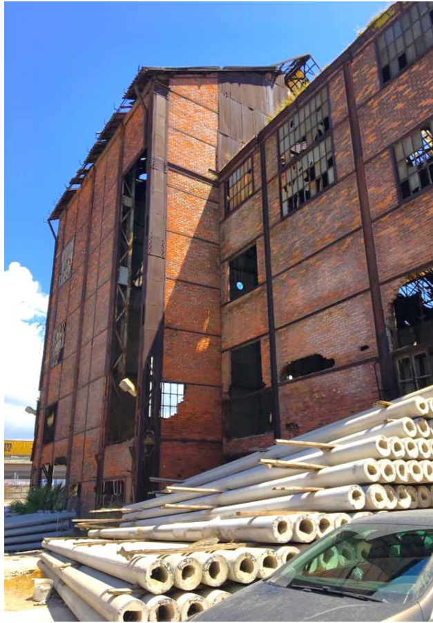
Fig 108: Photograph is taken by author during site visit
