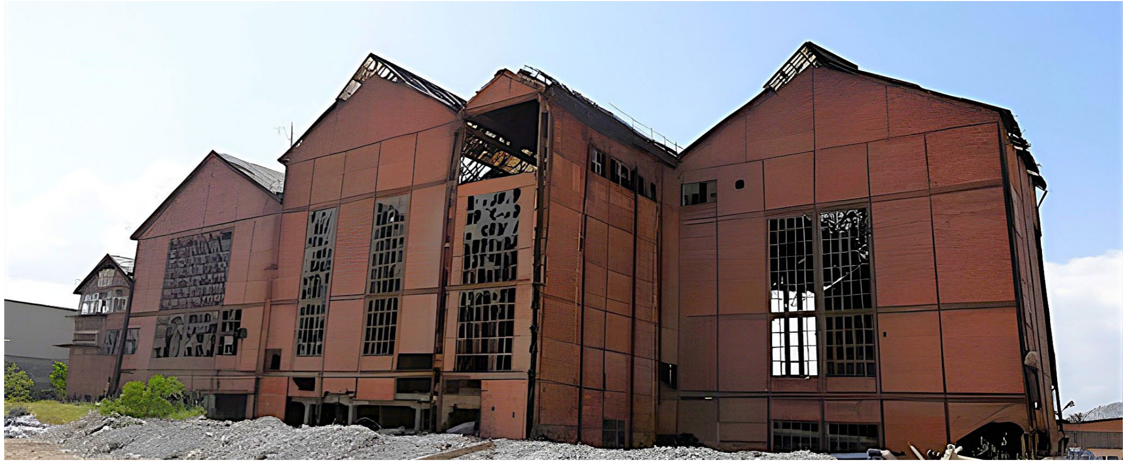
Fig 110: Photograph is taken by author during site visit
