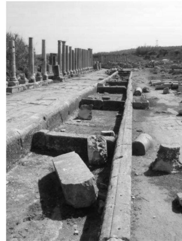
Figure 23. (a) Masonry channel with an open surface flow in the middle of Perge main street and with obstacles every 7 m. (b) Schematic top view of this channel, with the altitudes of some points/ Debaste, F., & Haut, B. (2014). Some elements of the water supply system of the city of Perge, in the Roman Imperial period, IWA Regional Symposium
