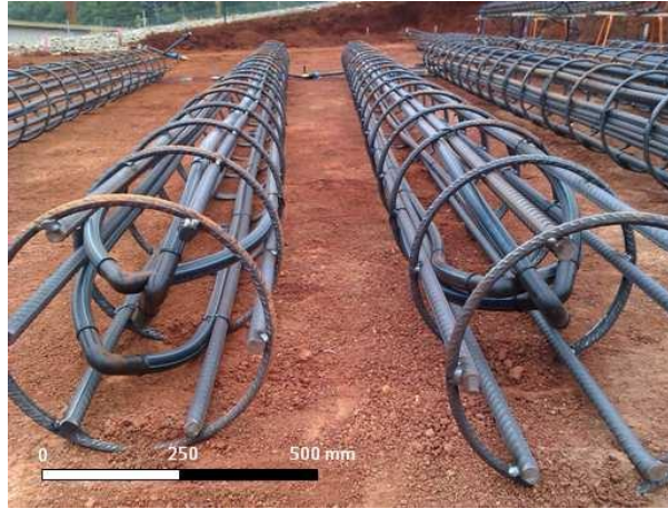
Figure 2-8. Fixed polyethylene pipes on the reinforcing steel cage of cast-in-place energy piles (Narsilio et al., 2014)
