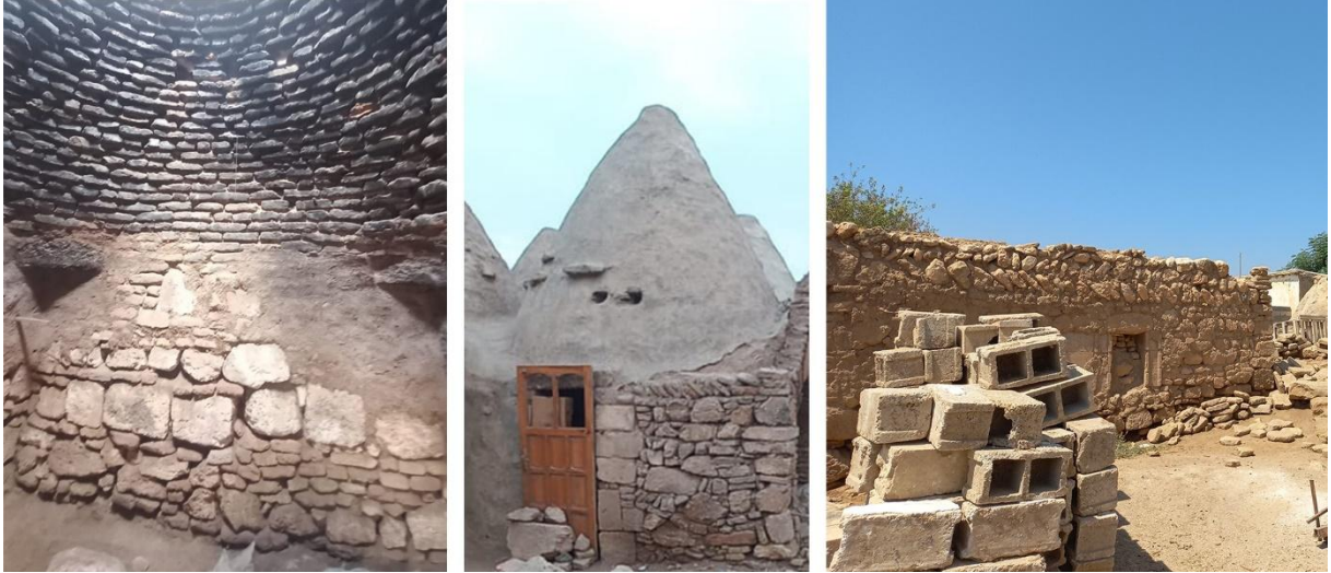
Figure 53 : From right to left, limestone and brick were used together in the first two photos. In the last photo, stone is the only material of the wall (2024).
