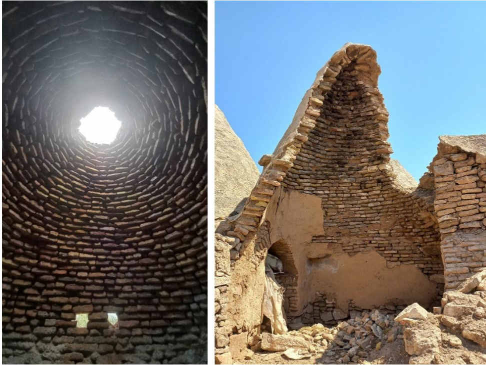
Figure 57 : The domes made of bricks of Harran houses, from left to right : bottom view of the dome, sectional view of corbelled dome of a collapsed house (2024).
