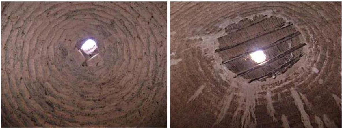
Figure 28 : Dome types of Suruç houses: conical dome (on the left) and flat-topped or truncated dome with wooden material used (on the right), (Şahinalp, 2012).
