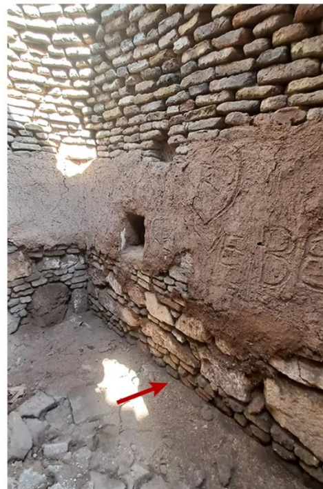
Figure 50 : Examples of combined use of different materials in the base. The red arrows indicate that the base begins with rows of bricks (2024).
