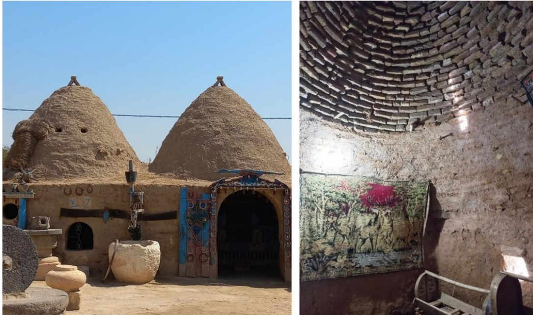
Figure 59 : From left to right : Completely plastered exterior surface, plastered interior walls and a partially exposed interior dome (2024).
