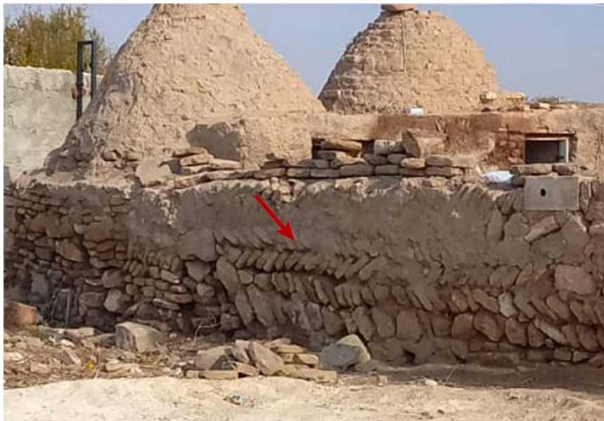
Figure 54 : An example of herring bone arrangement of bricks in the wall (2024).
