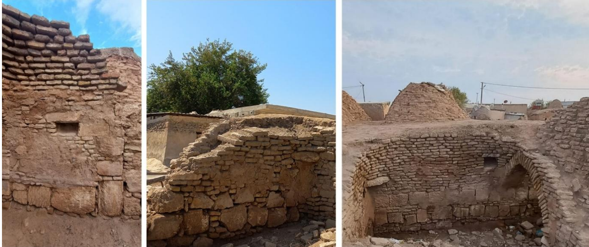
Figure 48 : Limestones used in the base of Harran domed houses (2024).
