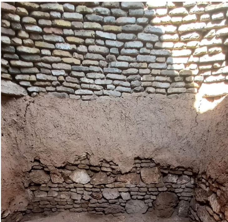
Figure 50 : Examples of combined use of different materials in the base. The red arrows indicate that the base begins with rows of bricks (2024).
