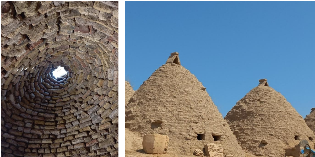
Figure 45 : Hole at the top of the dome in Harran houses (Harran, 2024).
