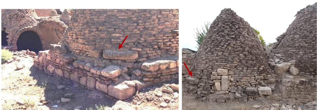
Figure 56 : Examples of Harran domed houses where the pendentive is visible from the outside. (From left to right: Tuncay, 2014 – Photograph by the author, 2024)
