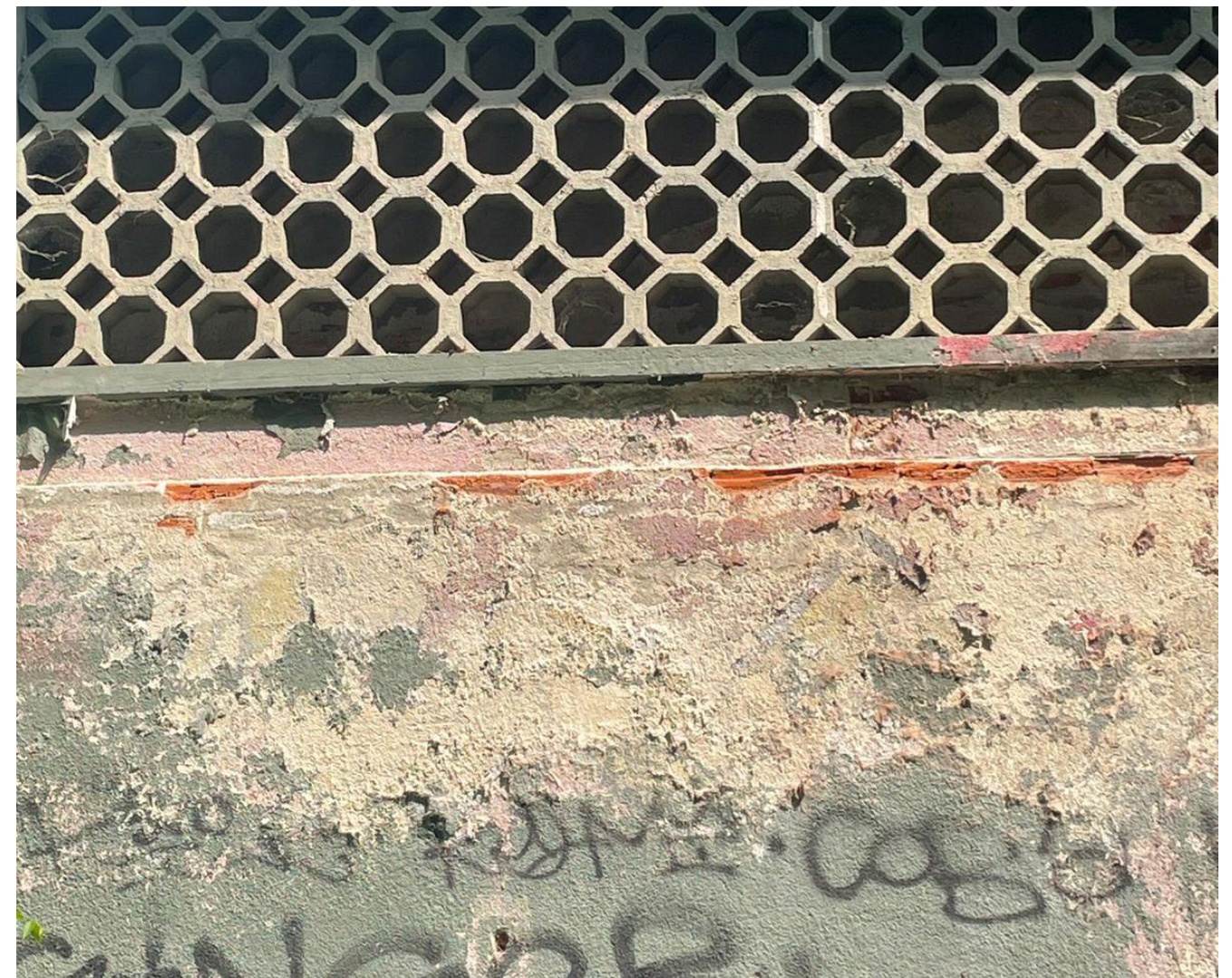
Figure 99: Pachyderm House - Delamination (Photo by the authors, 2025).
