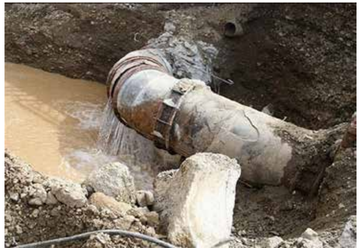
Water leakage due to wear and rusting of Tabriz water pipes
