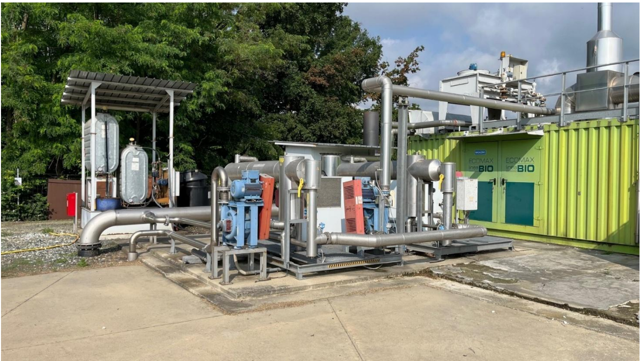
Figure 30 - Chiller for the biogas dehumidification.
