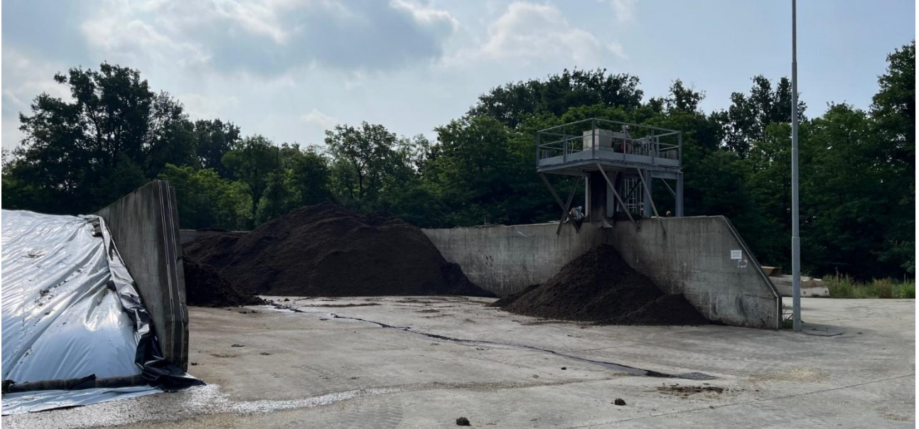
Figure 36 - Solid-liquid separator next to the digestate's trench.
