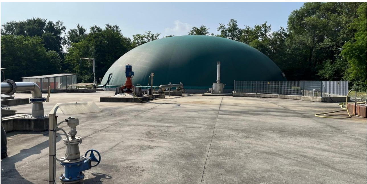
Figure 29 - La Falchetta plant with its gasometer over the third digester.
