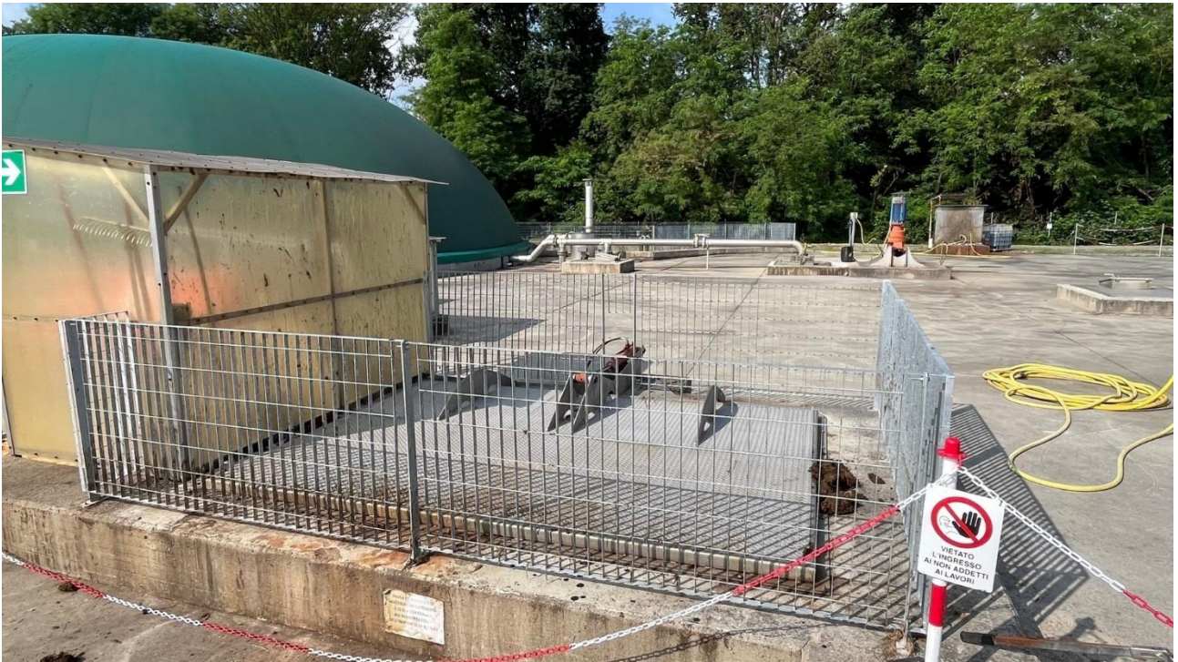
Figure 27 - Pre-tank for the liquid biomass storage and feeding.
