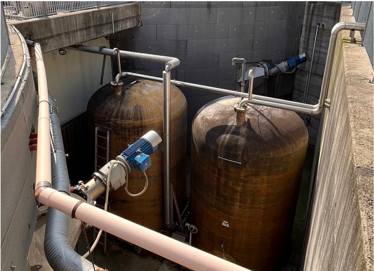
Figure 26 - Underground silos for the vinasse storage that will remain in operation.
