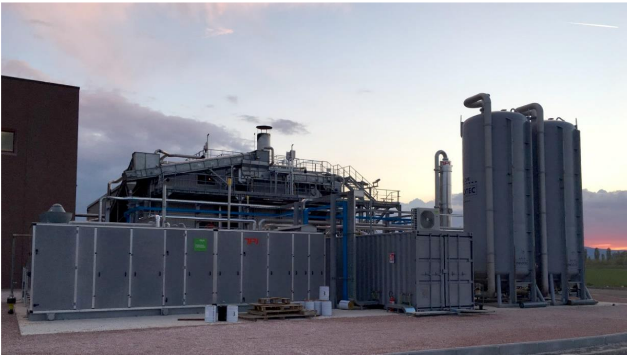
Figure 18 -Membrane upgrading unit in Foligno.
