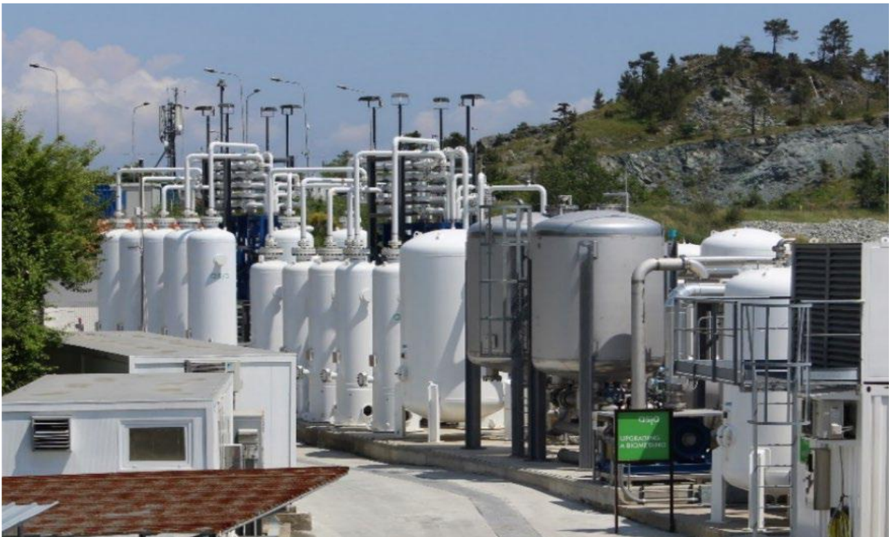
Figure 20 - PSA upgrading unit in Genova.
