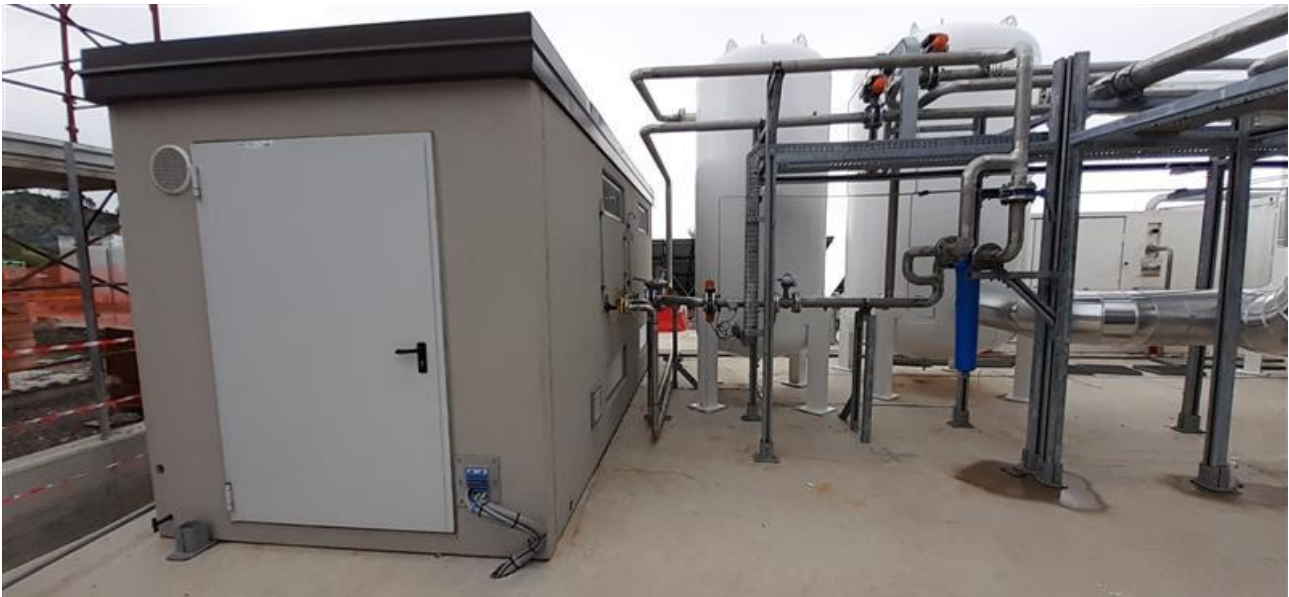
Figure 35 - REMI cabin station from Asja's plant in Genova.
