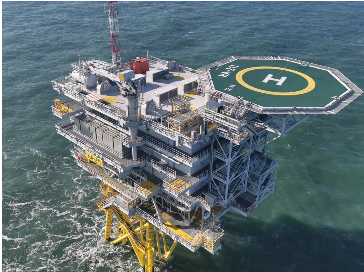
Figure 1.10: A fixed offshore substation, part of Hornsea One project
