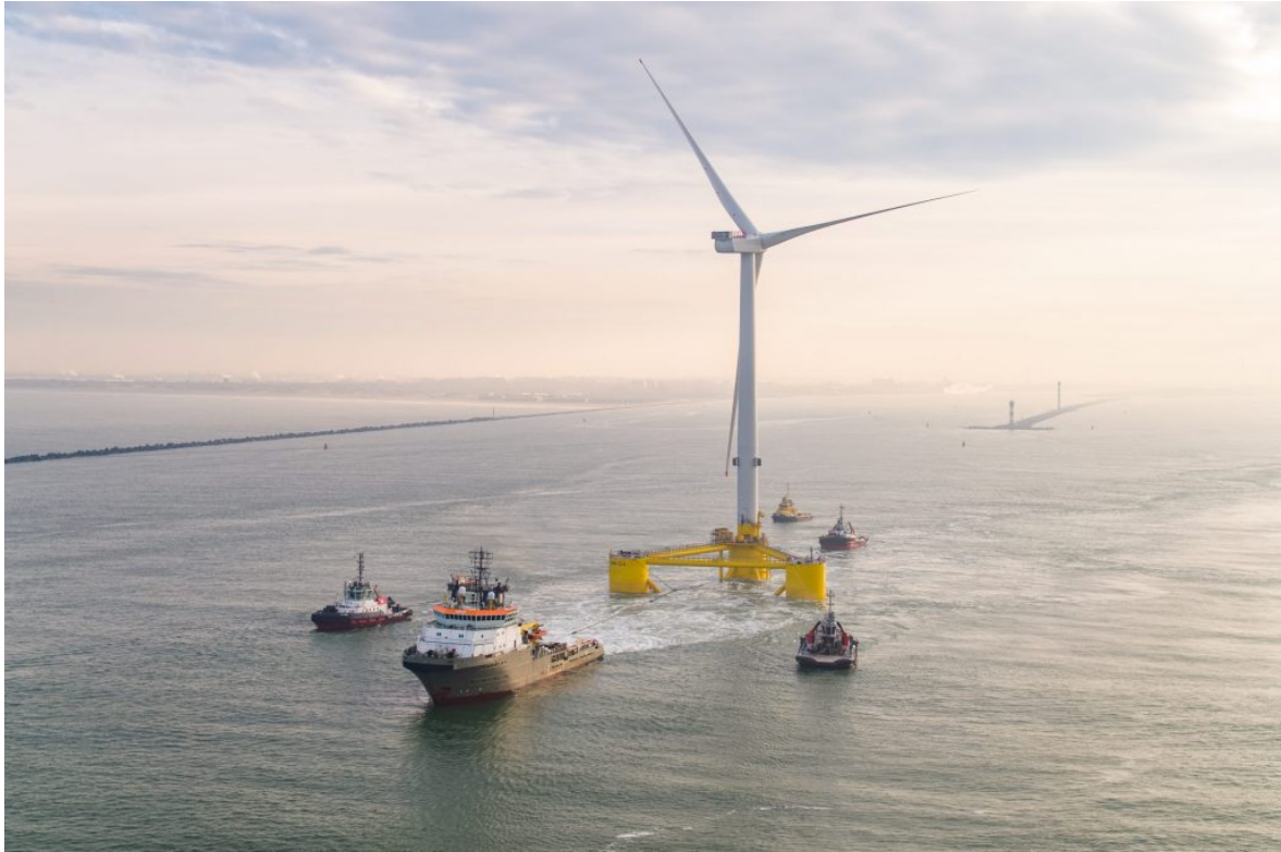
Figure 1.15: FOWT tow-out from Rotterdam to Scotland
