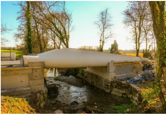
Figure 1.18: Two discarded turbine blades used to construct a bridge outside Cork City
