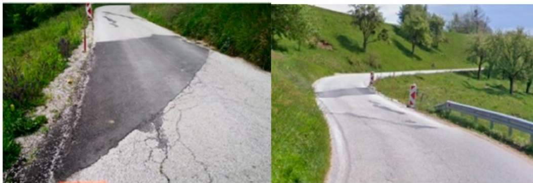
Figure 1 Landslides After Temporary Roadway Intervention, Source: Bračko et al. (2025)
