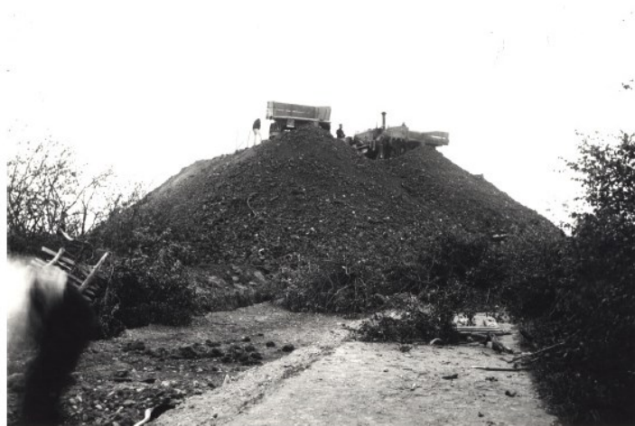
Figure 2 Image Showing End Tipping Construction Method Used in British Railway, Source: Walker et al. (2022)
