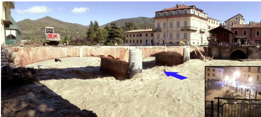
Fig. 11: Odasso Bridge. The light of the three arches has always proved to be insufficient for the outflow of the extraordinary flows, also due to the presence of considerable floating material. [1]
