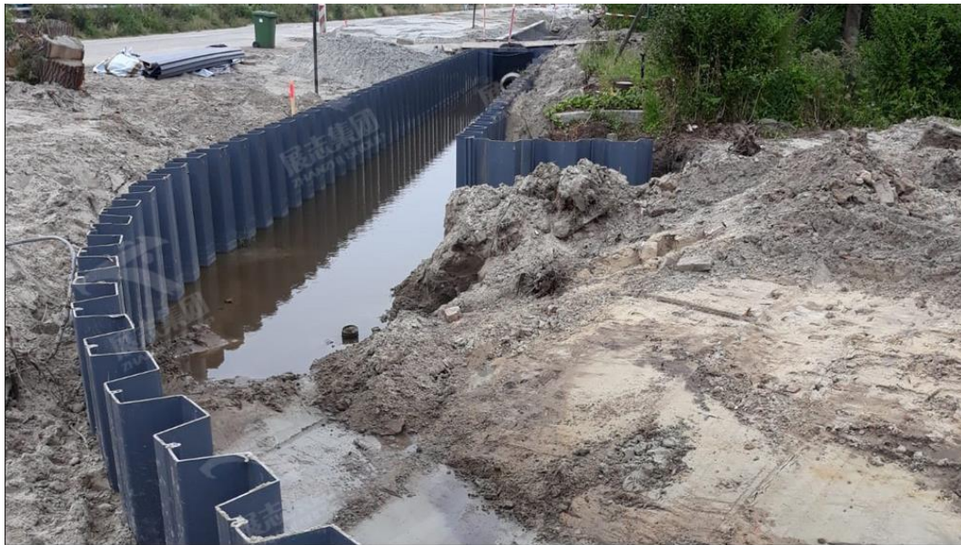
Fig. 28: Sheet piles positioned along a river. [72]
