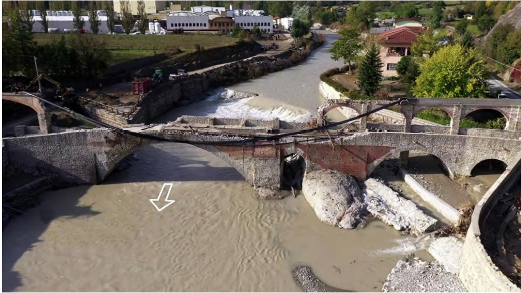
Fig. 9: Collapsed arches of the roman bridge in Bagnasco. [1]
