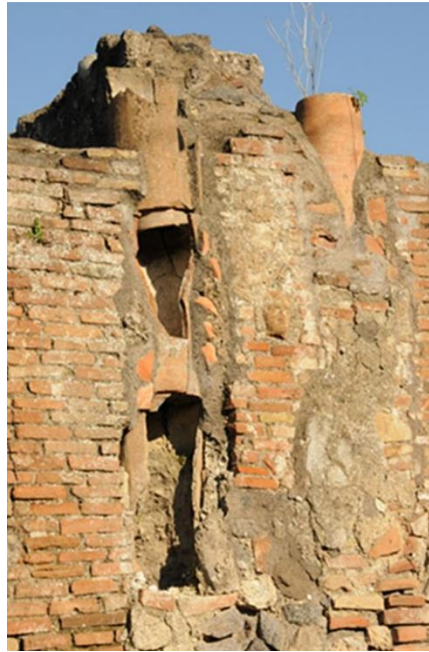
Fig 10. Terracotta pipe for rainwater harvesting from roofs at Pompeii, Italy. The pipes would have directed water into cisterns to service individual buildings(source: Charlesworth et al., 2016) .
