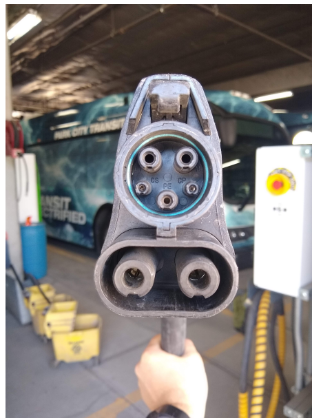
Figure 4.11: CCS-Combo 1 Connector used in North America
