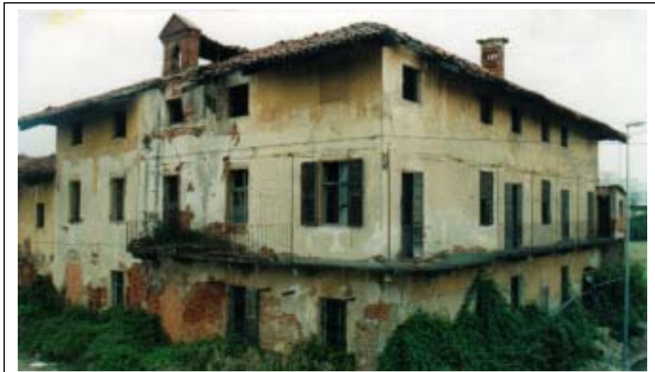
South-est view of the Cascina Borniola.
