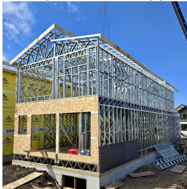
Figure 1.32: Roof trusses are lifted into place, completing the steel framing of a Cantiro home in Edmonton [10].
