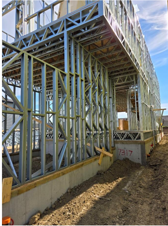
Figure 1.33: steel floor trusses allow for long spans [9].
