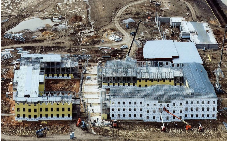
Figure 1.29: CFS-framed structure of Victory Hall at the University of North Texas [9].
