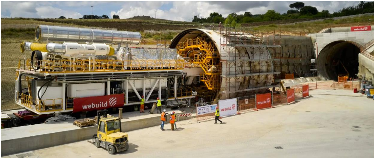
Figure 1.7 Assembly of conveyors for the Grottaminarda tunnel (Webuild)
