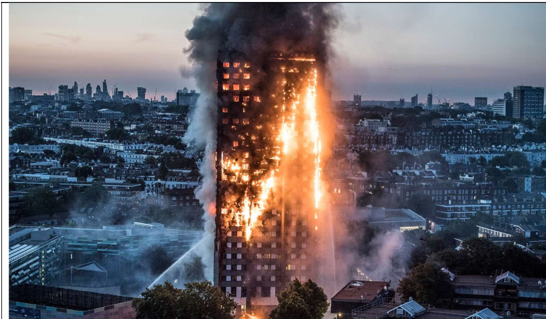
Figura 1 Incendio Grenfell tower [1]
