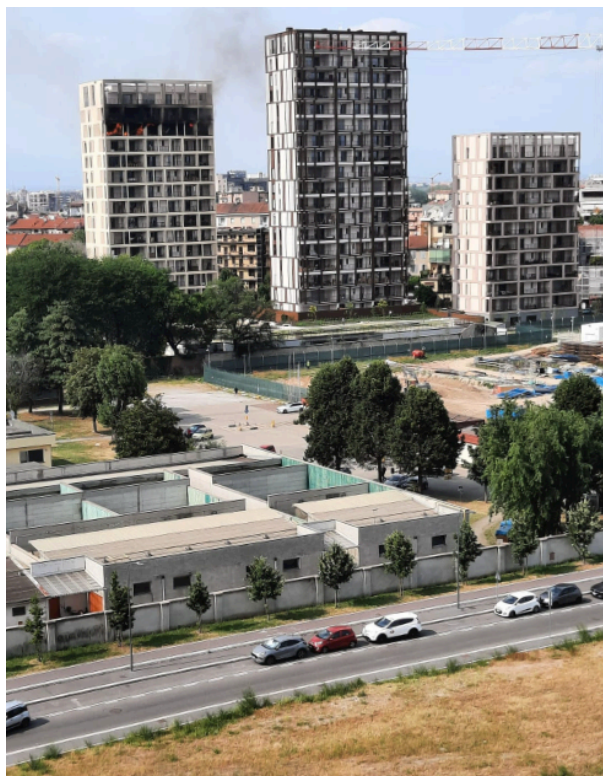
Figura 49. Complesso Trilogy Towers [62]
