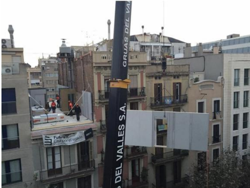
Figure 60 Lifting the prefab structure(Source: interempresas.net)
