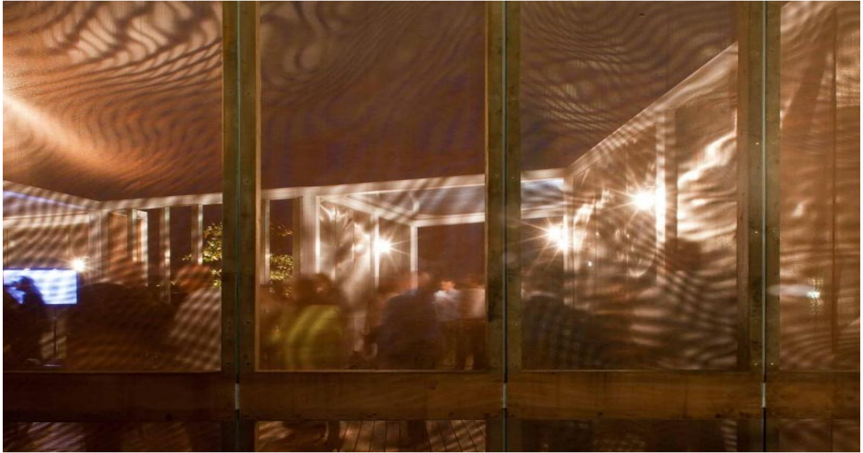
Figure 80 Copper and stainless steel mesh creates strong moiré patterns (Source: architecturefoundation.org.uk )
