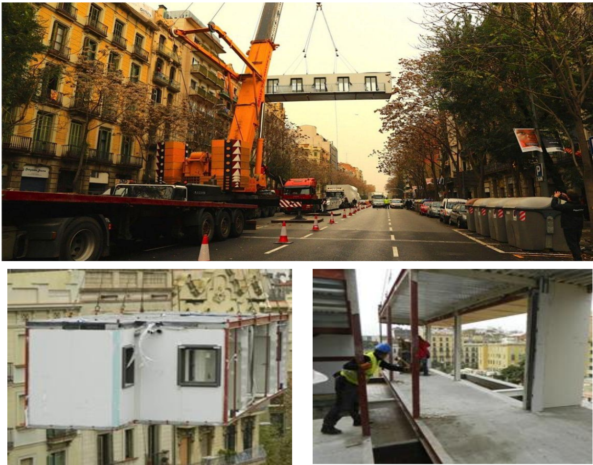
Figure 74 Pictures of the process of transportation and installation (Source: arquitecturayempresa.es )
