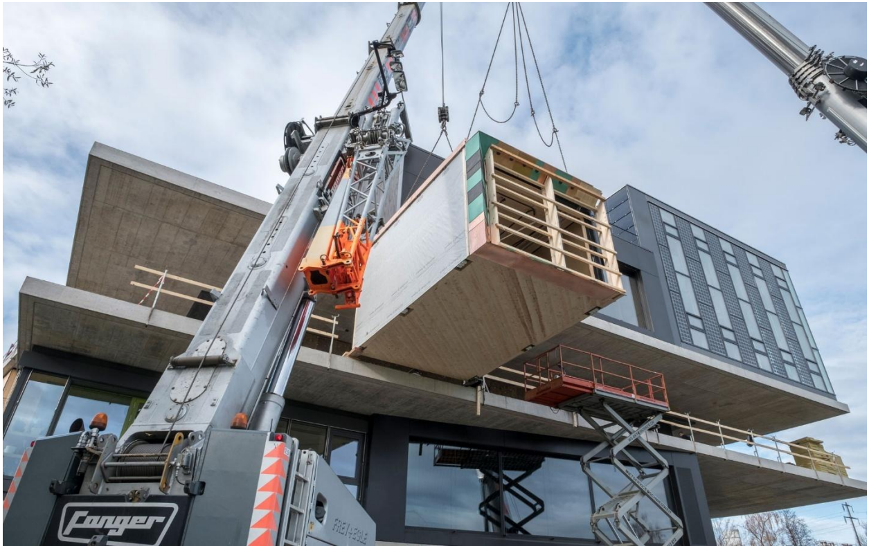
Figure 43 Lifting 3D modules over the rooftop
