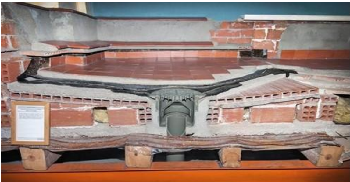
Figure 31 Picture of a model representing the Catalan Roof. The top part of this massive structure can be removed by hand to lighten loads of the building given that a new highly-insulated module will cover the building (source: La Casa por el Tejado)
