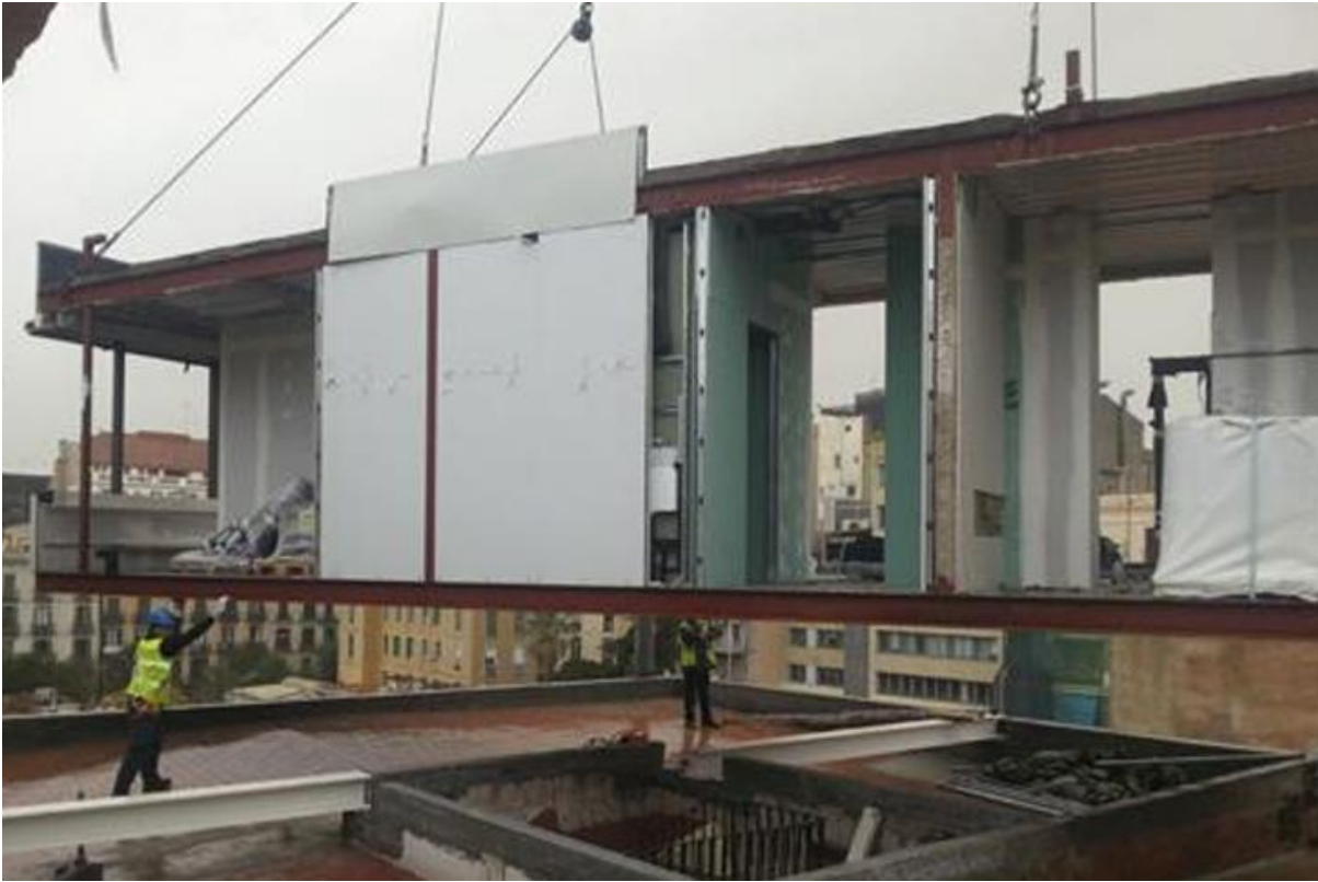
Figure 76 Picture of the central structural intervention on Aragó 359: the chained forged beam is seen at the bottom of the picture
