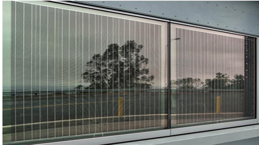
Figure 109 Building Integrated Photovoltaic (BIPV) window
