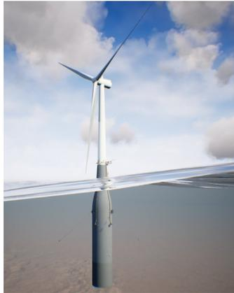
Figure 2.3: Spar-type platform Hywind by Equinor [6]
