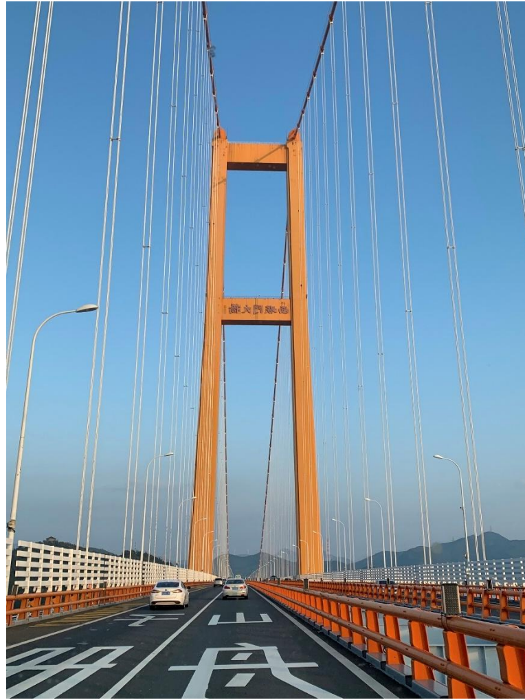
Figure 3.8 - View of hangers and the north pylon[21]
