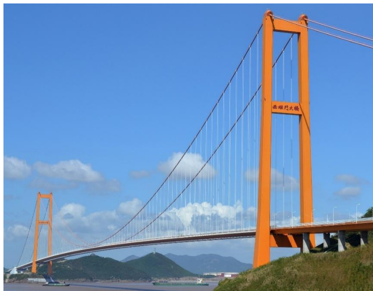
Figure 3.3 – Overview of the Xihoumen Bridge[18]
