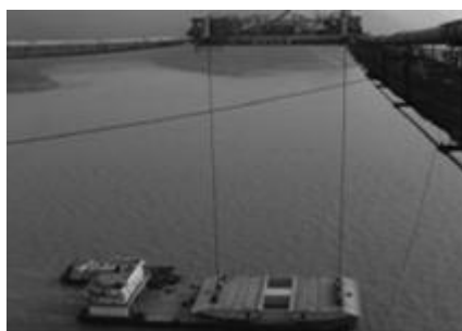
Figure 3.7 - Dynamic positioning of carrying boat[19]
