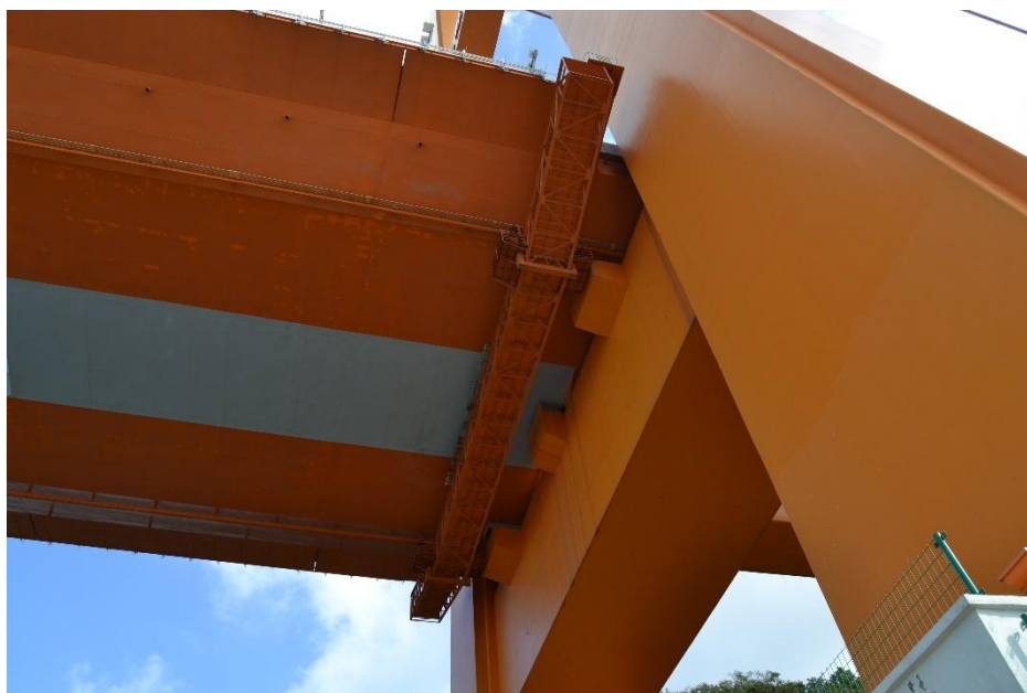
Figure 3.10 - Particular of cross beam of south pylon[18]
