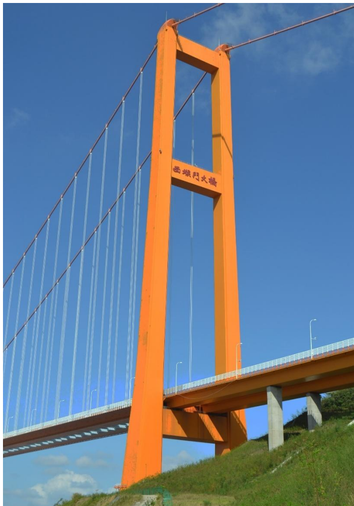
Figure 3.9 - View of south pylon[18]
