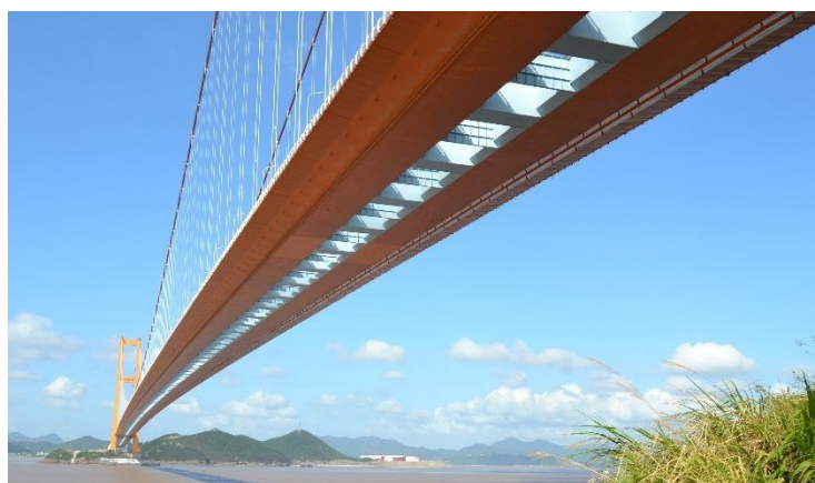
Figure 3.5 - Particular of the twin-box girder deck[18]
