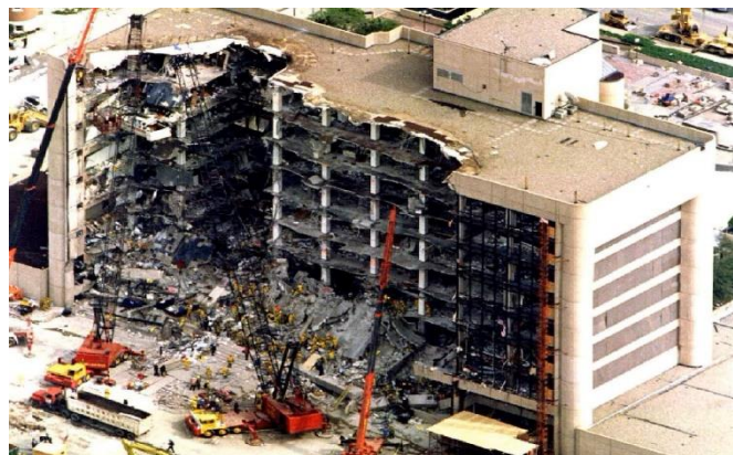
Figure 2: Esplosione del Murrah Federal Building ad Oklahoma City (1995).
