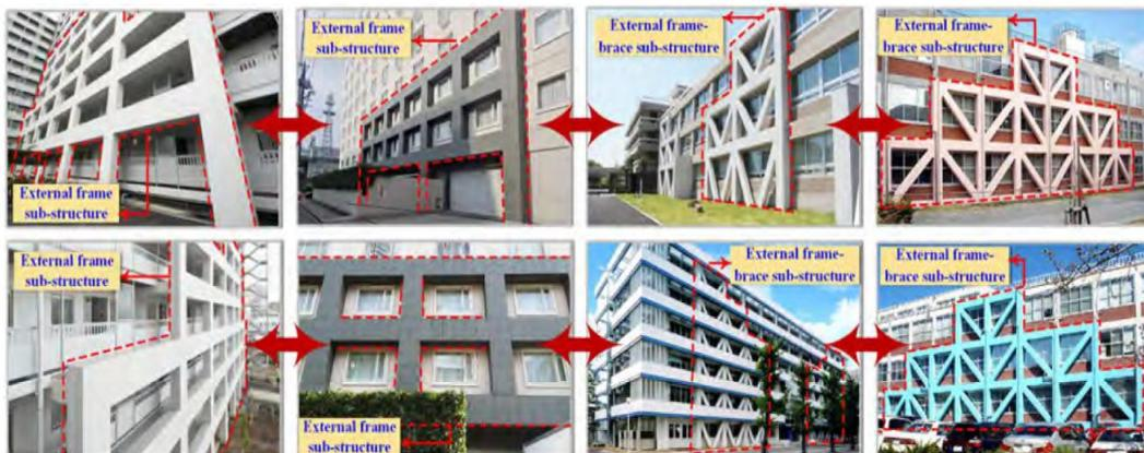
Figure 1: The typical cases of the external sub-structure retrofitting method [1].
