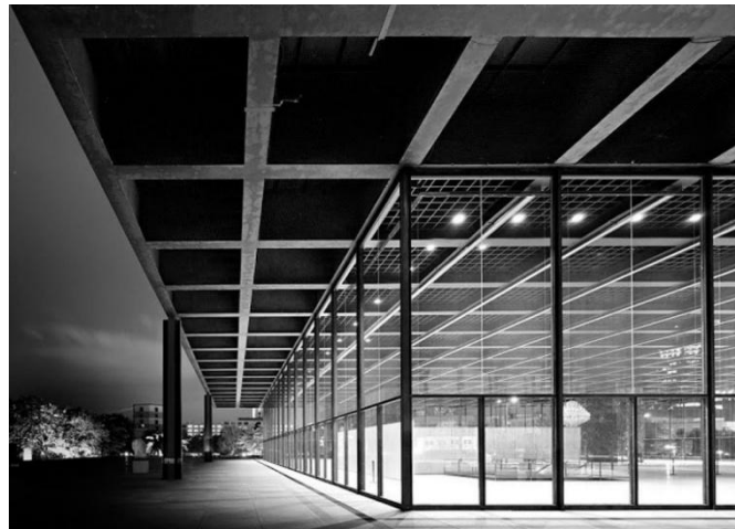
Figure 2-8: Details of the glass façade and the suspended roof of the Neue Nationalgalerie 9 .
