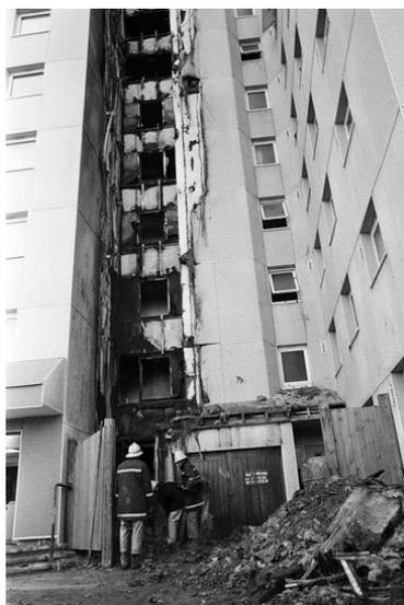
*Figura 72 - Esempio rientranza (Liverpool Echo) (Peacock, THE RELATIONSHIP BETWEEN BUILDING DESIGN AND FIRE SPREAD: How the shape, form and features of a building can influence the behaviour of fire, October 2019 )*
