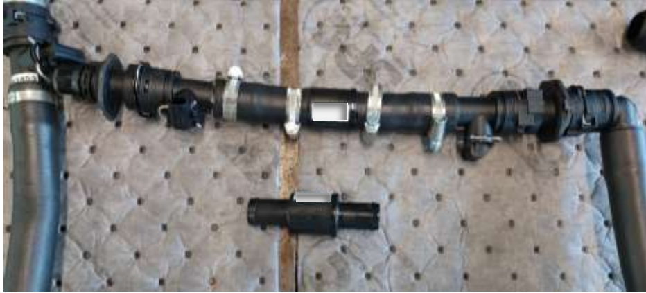
Figure 2-3: Valve and pipes setup
