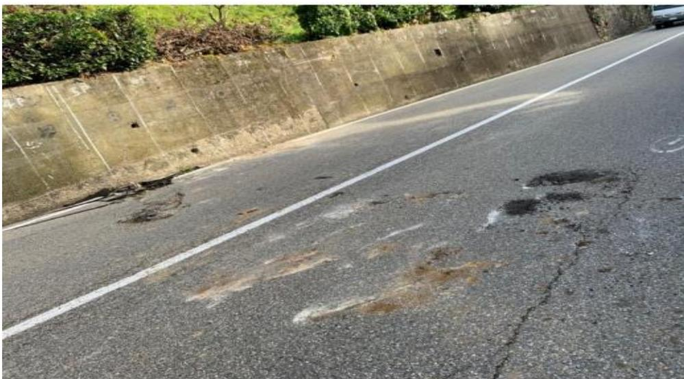
*Figure 3.1.3.2 damage to the road surface by rockfall*
