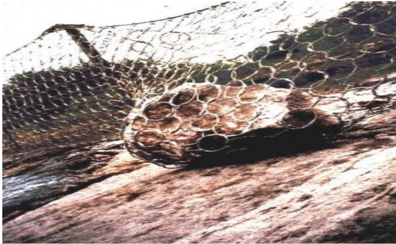
*Figure 2.3.1.9.1 Geobrug ring net shown restraining a boulder. These nets can be designed with energy absorbing capacities of up to 2500 kNm which is equivalent to a 6 tonne Boulder moving at 20 m per second*
