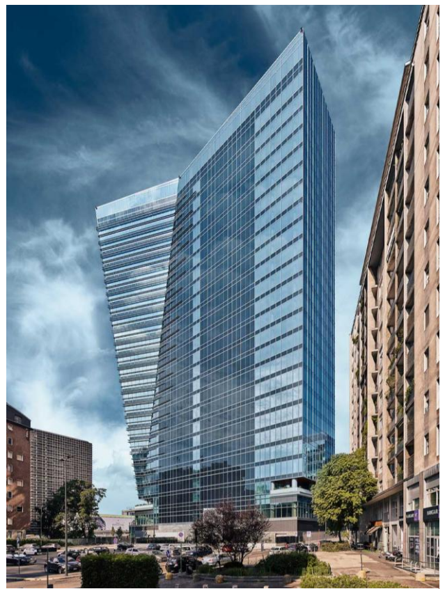
Figure 47. Gioia 22 with BIPV Adaptive Facade, Milan
