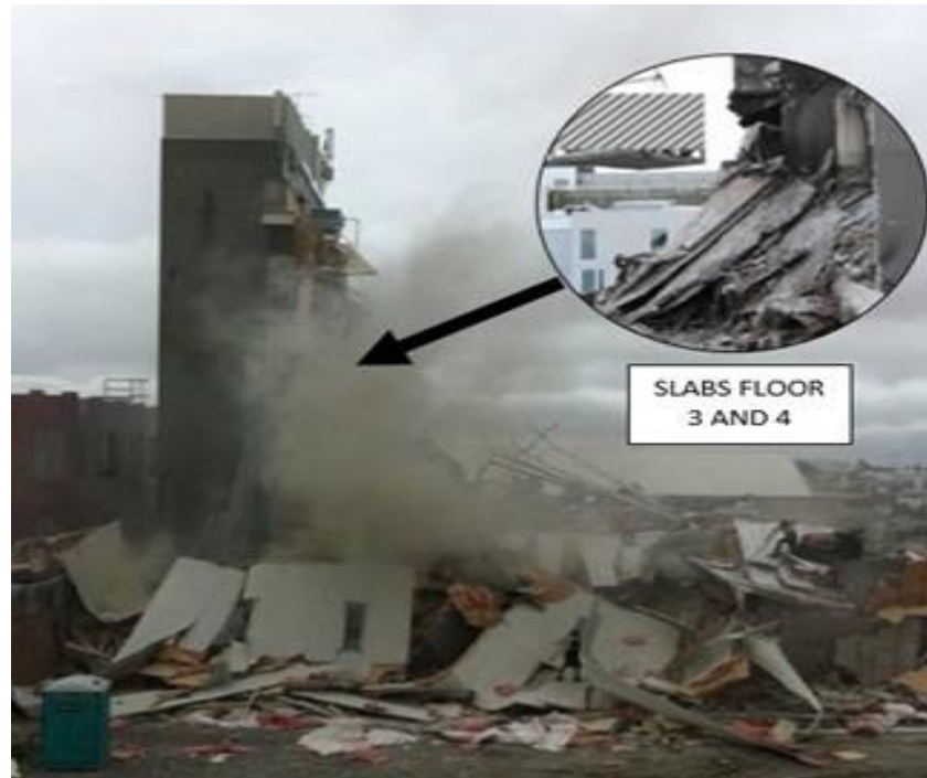
Figure 26 - ( 2011 Christchurch Earthquake ,New Zealan) The CTV Building in Christchurch collapsed due to vertical irregularities. The building had significant stiffness changes between floors and inadequate lateral load resistance, which led to a catastrophic failure when subjected to earthquake forces
