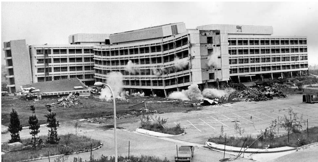
Figure 24 - Olive View Hospital (California, USA – 1971) Severely damaged in the 1971 San Fernando earthquake (M6.6) due to horizontal irregularity
