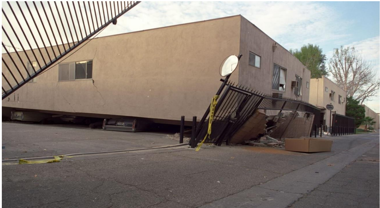
Figure 29 – ( 1994 Northridge Earthquake ,Los Angeles, USA) The Northridge earthquake exposed the vulnerability of soft-story apartments, especially in multi-story residential complexes. Many buildings with open parking spaces on the ground floor collapsed, including the Northridge Meadows apartment complex, where the soft-story failure led to multiple fatalities. The destruction prompted stricter building codes and retrofitting initiatives in seismic-prone regions
