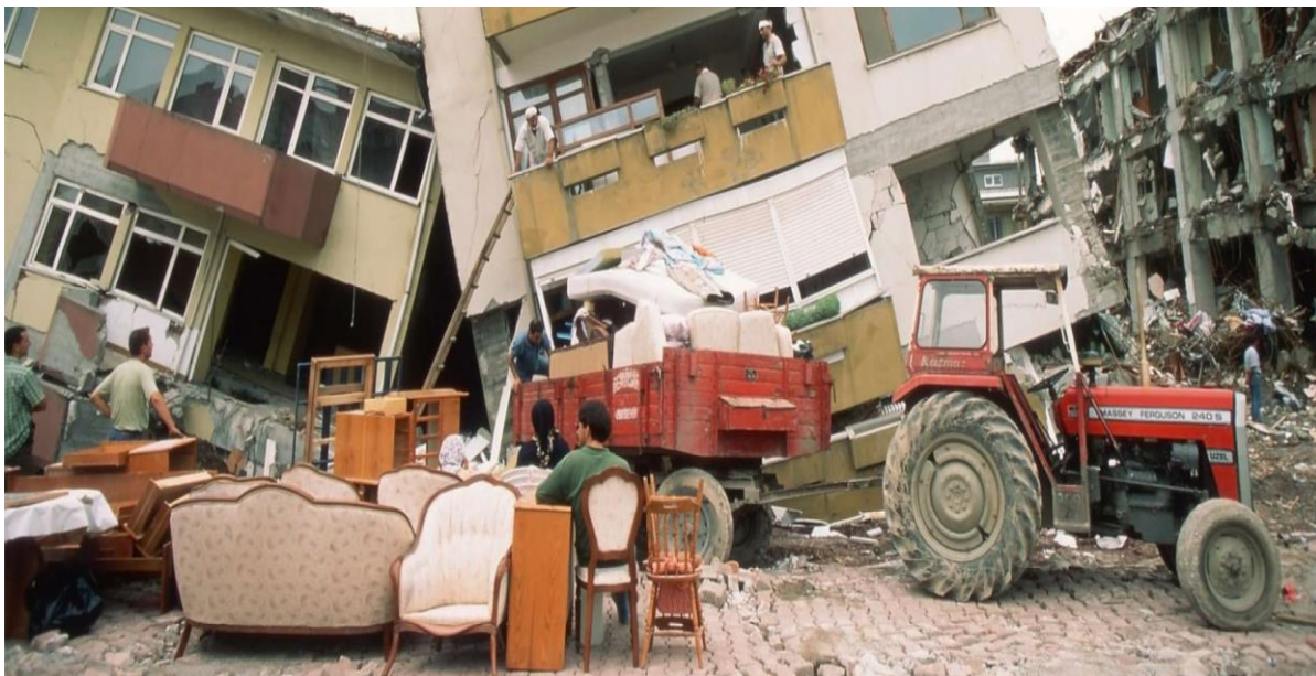
Figure 31 – ( 1999 İzmit Earthquake , Turkey)In the 1999 İzmit Earthquake, multiple buildings constructed in close proximity were severely damaged due to the pounding effect. The destruction was most evident in older, poorly designed structures, where unreinforced concrete walls and columns suffered significant cracks and failures due to repeated collisions with neighboring buildings
