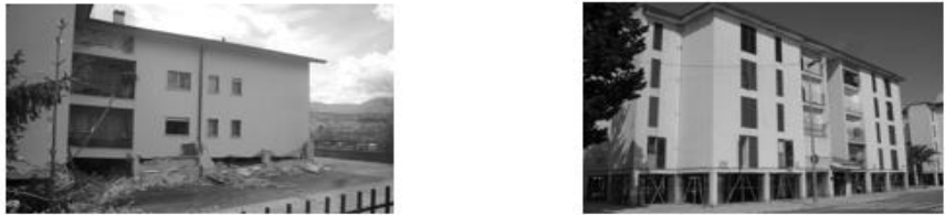
Figure 2.5. Two recent examples of severe damage attributed to the soft first story irregularity in L'Aquila earthquake, Italy in 2009, (Photos, left: Holly Razzano, Degenkolb) and in Lorca, Spain in 2011.
