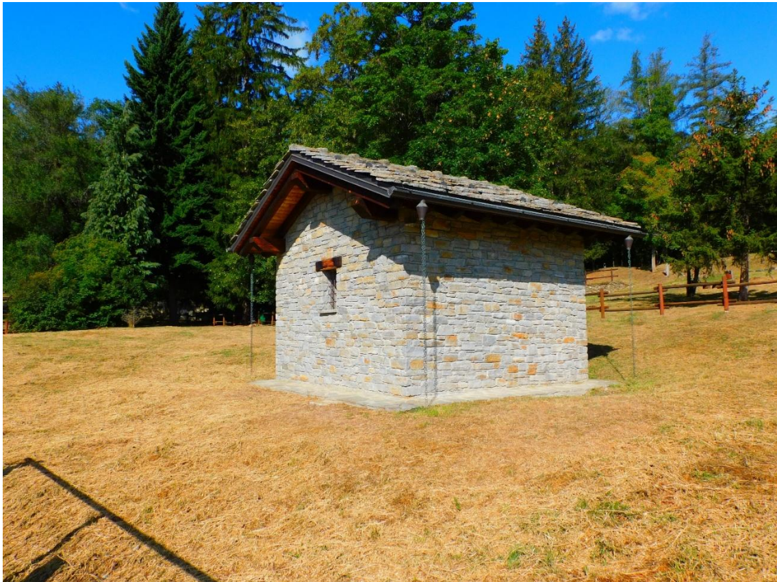
Figure 5 - Monitoring infrastructure housing the spring and associated instrumentation for hydrological data collection.
