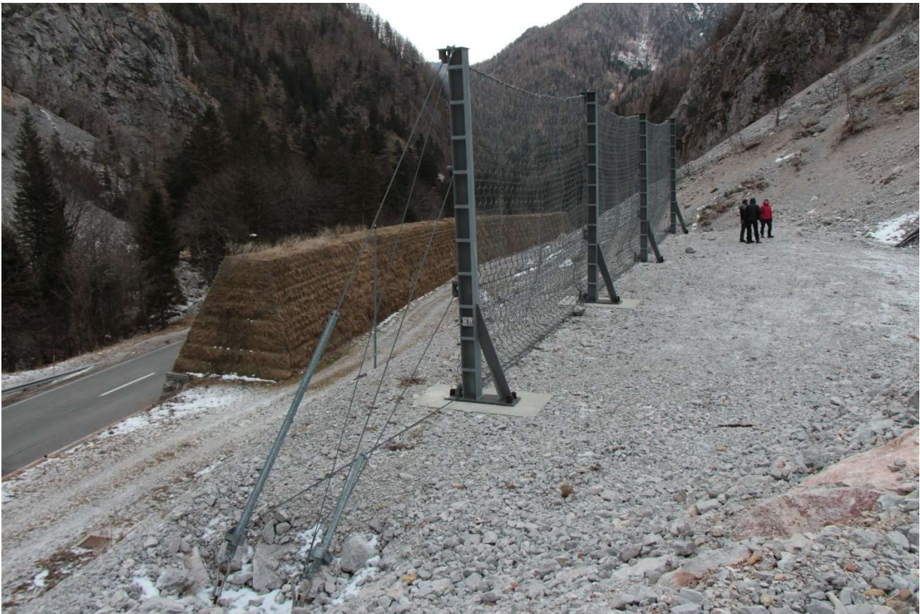
Figure 5-3 Embankment and net fences against rockfall about 300 metres north of the Podljubelj tunnel (Photo: Miha Pavšek, ZRC SAZU)
