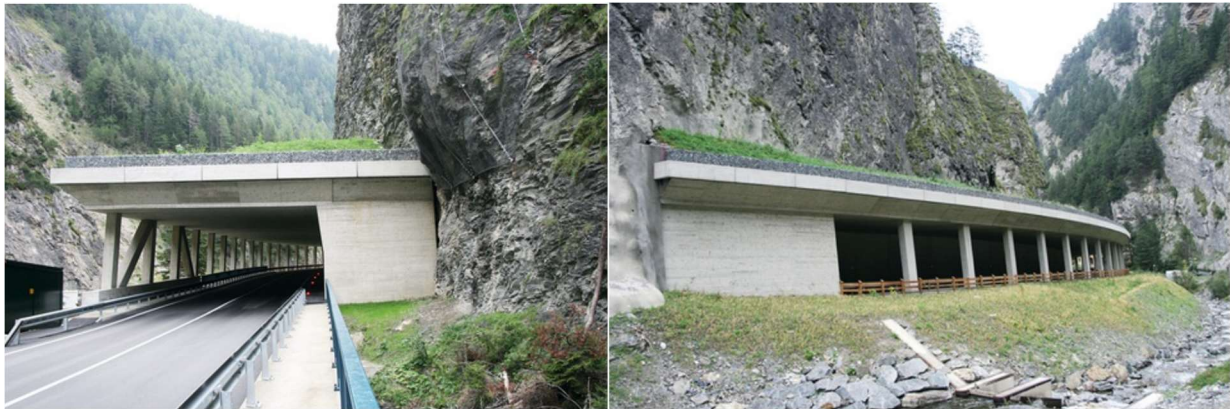
Figure 6-2 Left: Nauders gallery portal. Right: Connection of gallery structure with natural tunnel. (Source: PORR AG)
