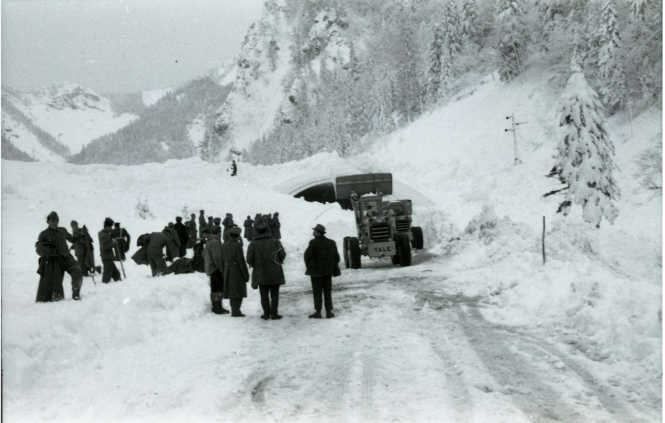
Figure 5-10 Removal of snow obstructing the tunnel entrance. Estimated period 1965 (Source: SNEŽNI PLAZOVI I. DEL dipl. inq. Jože Pintar, Podjetje za urejanje hudournikov Ljubljana, 1968)
