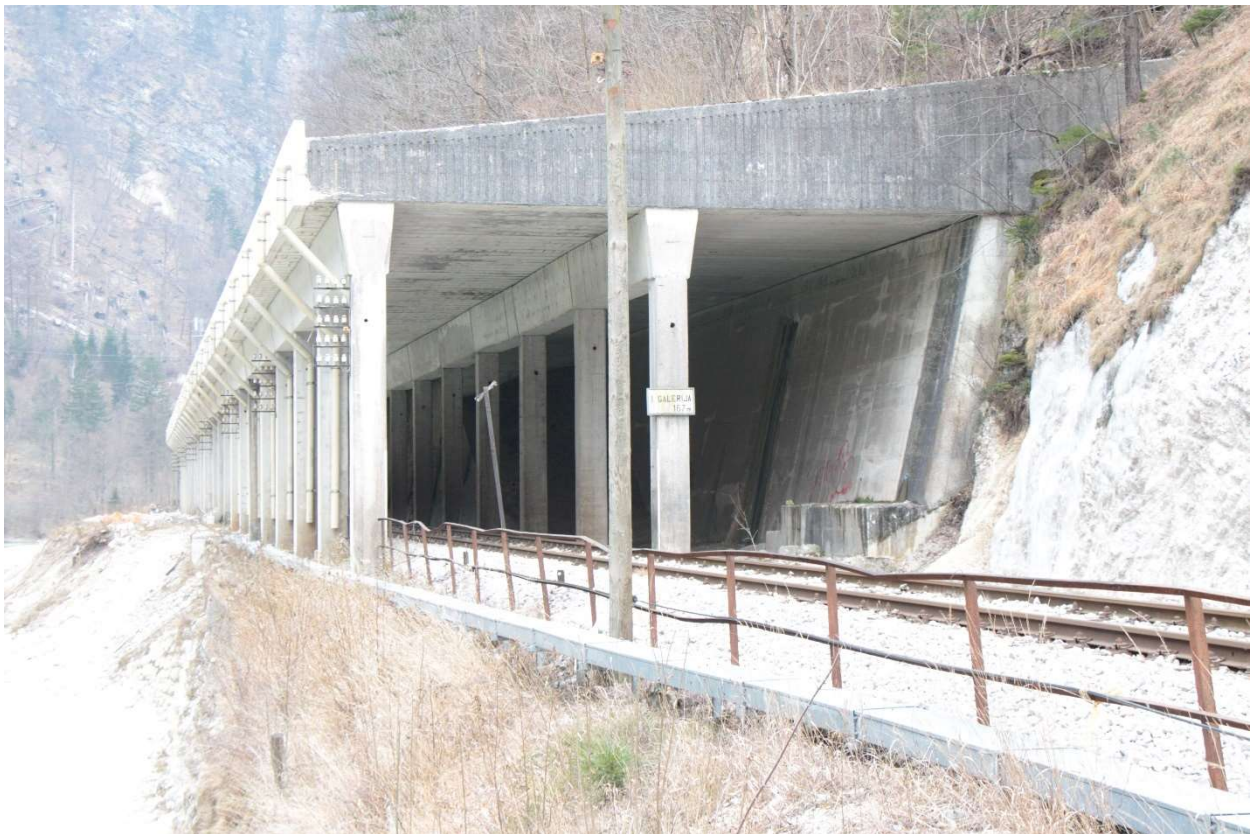
Figure 3-5 Avalanche tunnel, Slovenia (Photo: Miha Pavšek, ZRC SAZU)
